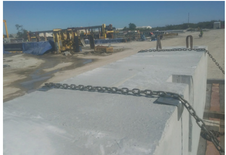
Correct strapping with chain guards
