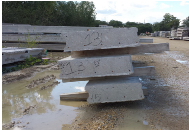
Misaligned stacking, tilted stack, and soft ground
