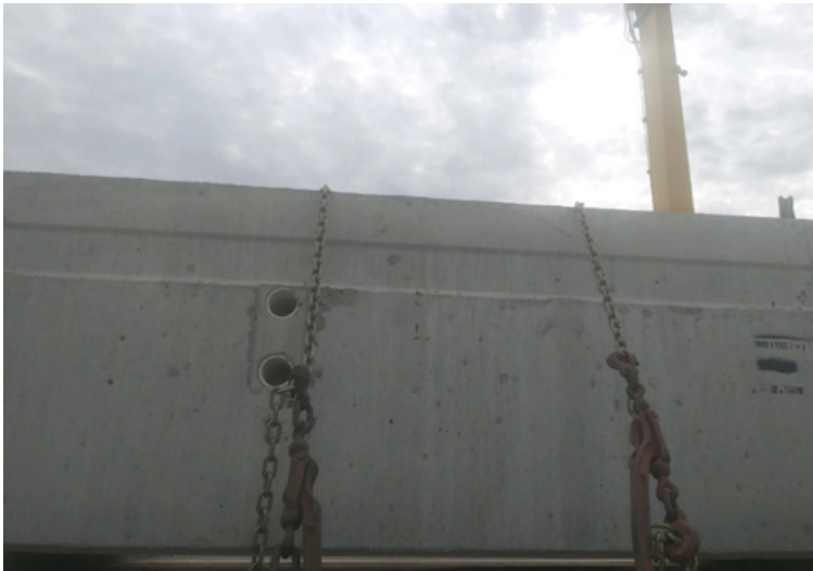
Incorrect strapping without chain guards
