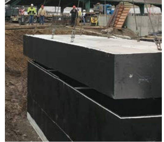
Photos courtesy of Kistner Concrete Products Inc.
