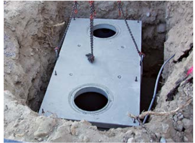
Photos courtesy of Jensen Precast
