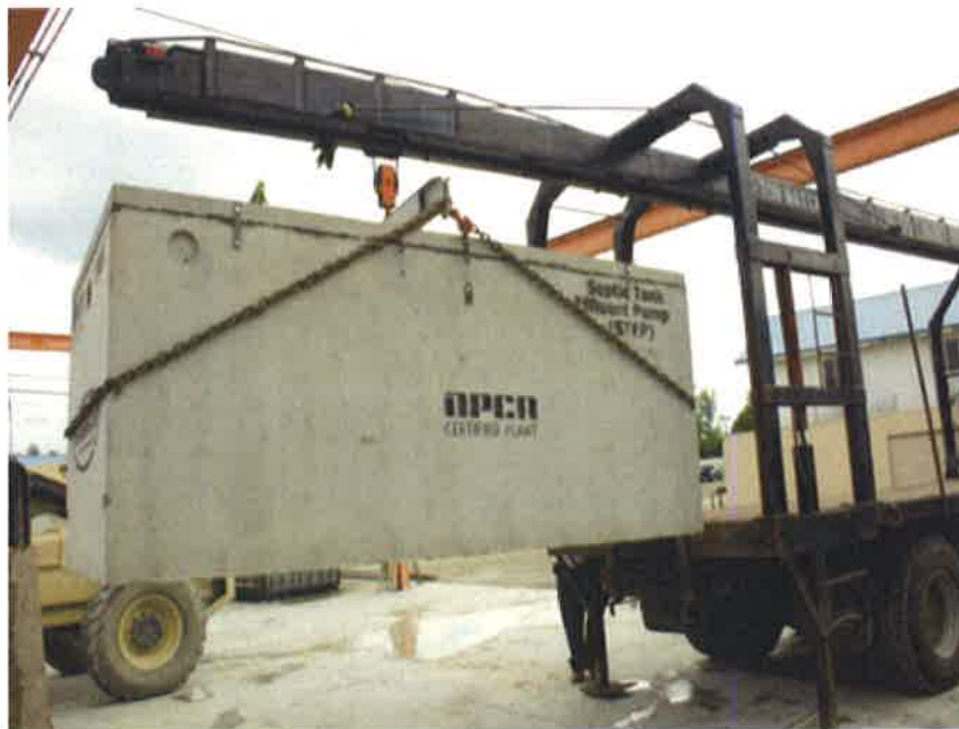
Photo 3: Septic Tank Delivery Rig
