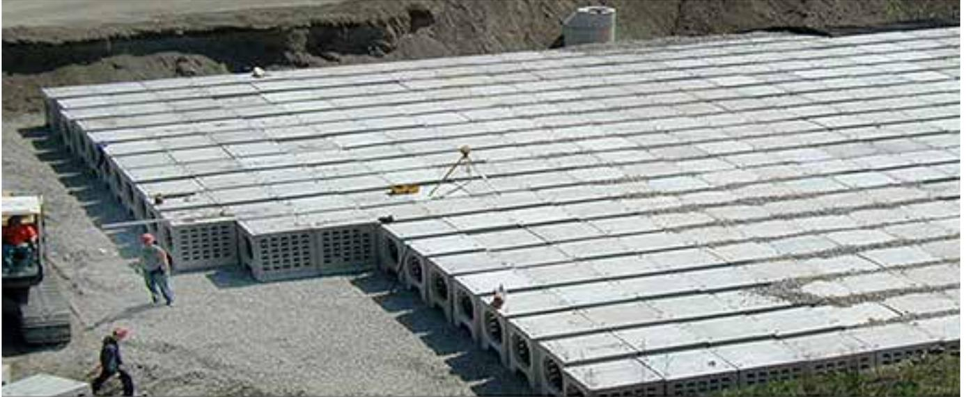
Any grouting that will inhibit the design/flexibility of the connector should be avoided.
