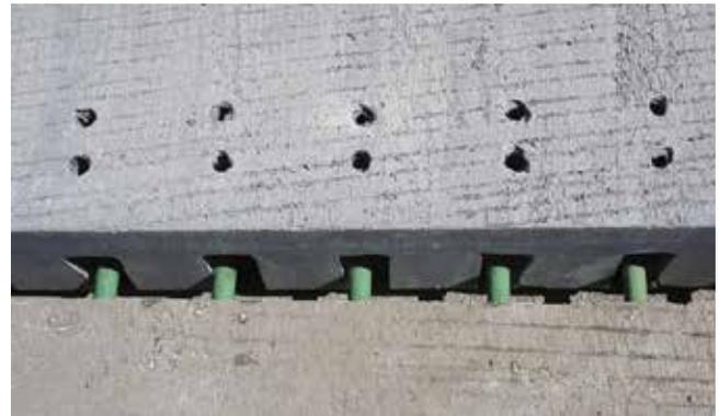
Figure 12: Installation of bottom slot Super Slab® system.
