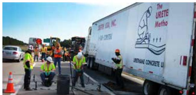
Figure 9: Urethane installation for the Roman Road system.
