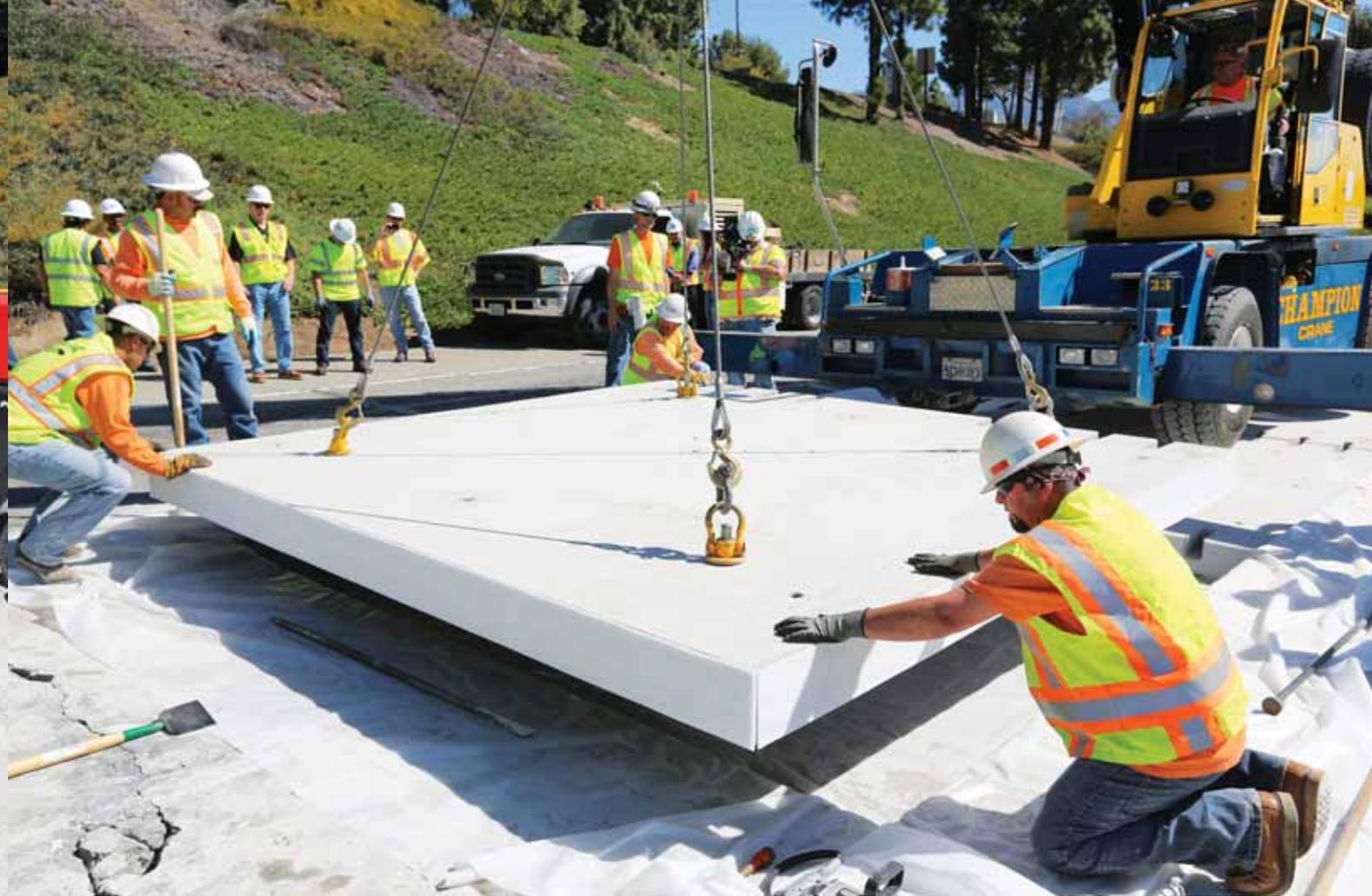
bridges for decades—now its time in roadway reconstruction apparently has come. The I-710 project involves 36 lane-miles of concrete panels, equivalent to 831,000 sq ft or 27,700 cu yd. Among the application's various challenges is the fact that, because of the roadway's geography, the panels taper in width from 26 ft on one end to 36 ft on the other. "Each panel has to get slightly larger so each one is different," Stahl said.
