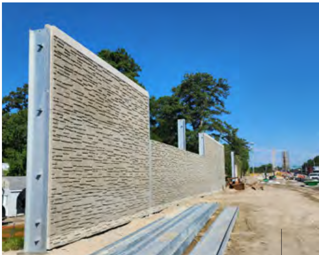
Smith-Midland is producing approximately 170,000 square feet of absorptive sound wall for the Hampton Roads project.
