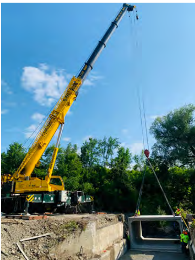
LHV manufactured the replacement of the culvert bridge on County Route 32 in Otsego County, N.Y.
