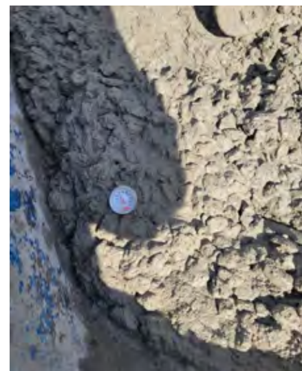
Thermometer in fresh concrete
