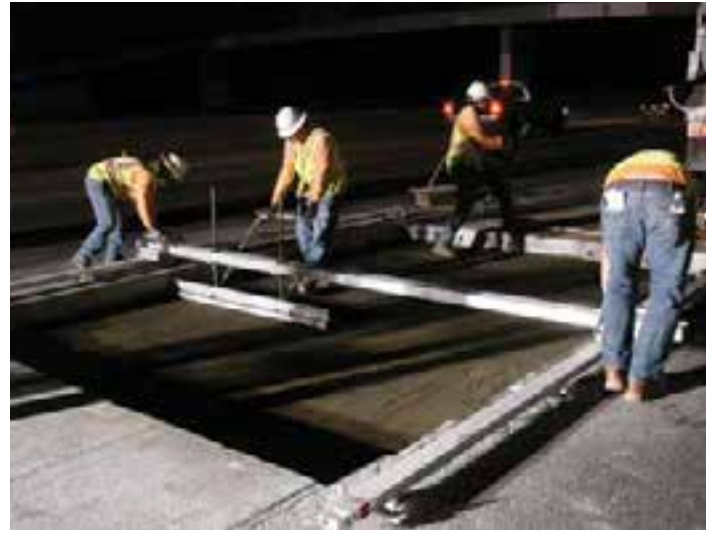
Figure 10-13. A four-man crew grading fine aggregate bedding material.
