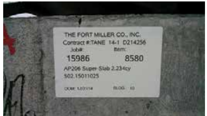
Figure 7-28. Example panel label showing all the information needed for identification purposes.
