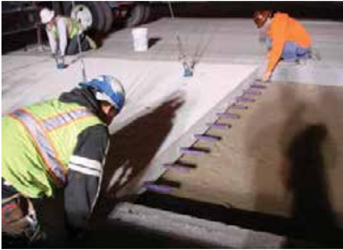
Figure 9-52. A PCP panel being placed to a leading end line stretched between two leading end marks.
