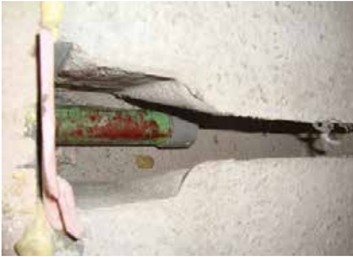
Figure 9-34. The hole drilled for the dowel in this photo was not closely aligned with the cast-in slot, making dowel installation difficult.
