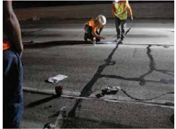
Figure 8-10. Workers using a right-angle laser tool to accurately mark a perpendicular transverse saw cut for a straight roadway.
