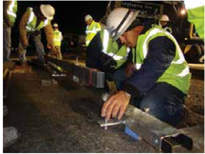
Figure 10-7. A grading crew checks and adjusts screed rails to ensure an accurate grading frame of reference.
