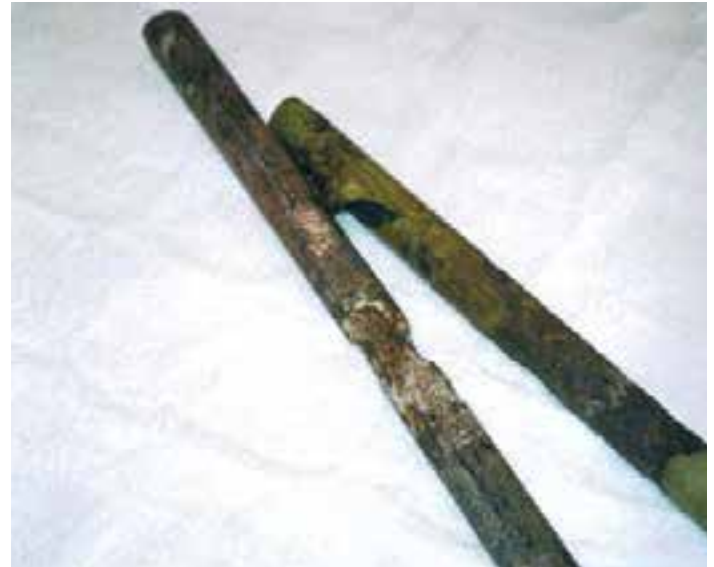
Figure 4-24. Dowels retrieved from Minnesota pavements after 17 years or more of service.
