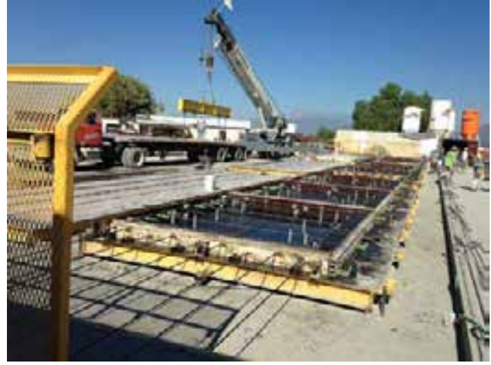
Figure 1-9. Photo of JPrCP fabrication in a prestressing bed.
