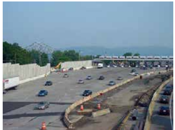
Figure 3-21. The expanded Tappan Zee Bridge toll plaza after precast panel installation was completed in 2002 (photo taken during off-peak hours to highlight the expanse of precast panels).
