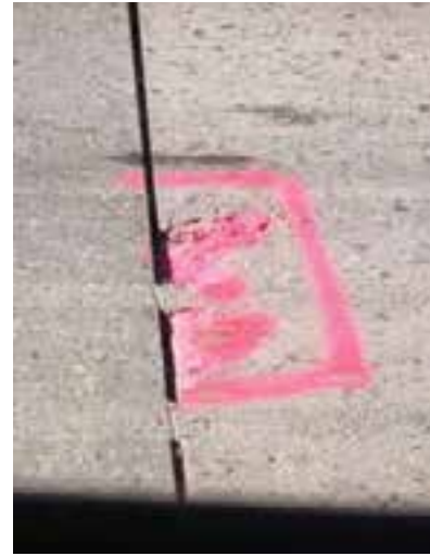
Figure 11-4. Photo showing failure of backfill material in top slots around the dowels and failure of the concrete between the slots.
