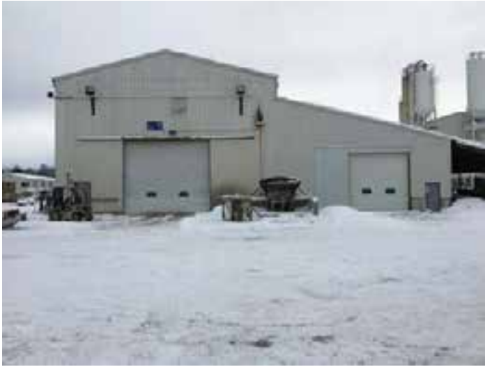
Figure 7-1. An insulated, temperature-controlled building allows casting in all types of weather.
