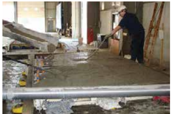
Figure 7-20. Concrete placement directly from a ready-mix truck (form is low enough to permit direct placement from the truck).
