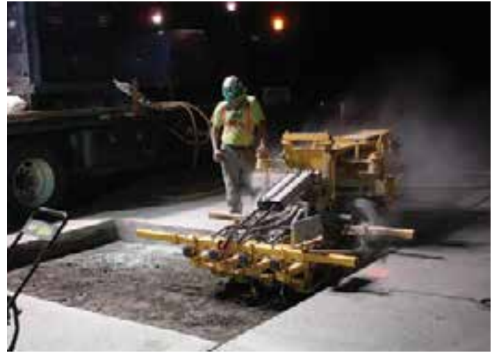
Figure 9-24. This gang drill is capable of drilling four holes at once in approximately 20 to 30 seconds.
