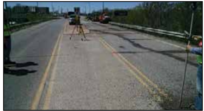
Figure 6-6. Collection of existing pavement data using a robotically controlled total station.
