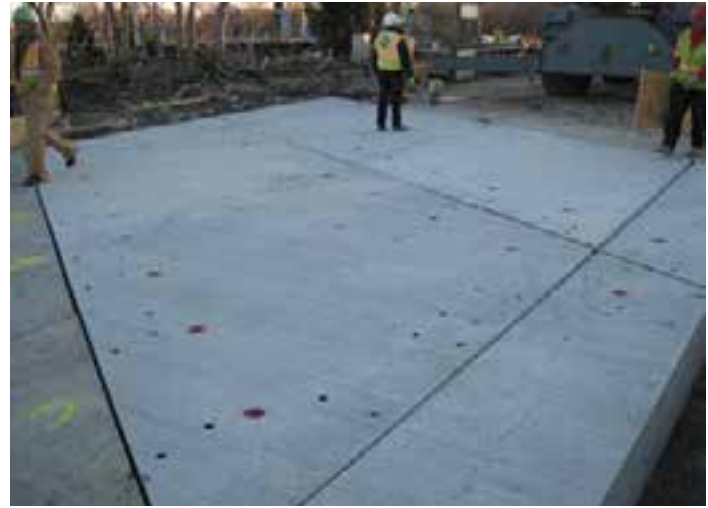
Figure 3-23. New precast concrete bridge approach panels at the Route 46 Bridge in Clifton, N.J.
