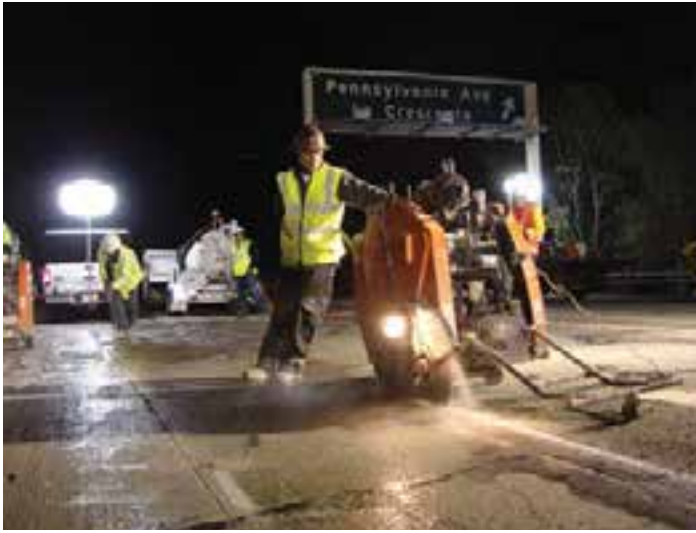
Figure 10-12. A sawing crew consisting of two saw operators and one slurry cleanup man.
