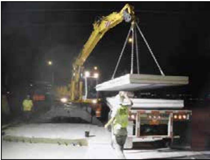
Figure 6-4. Rubber-tire excavator placing a 12-foot-wide-by-10-foot-long panel. The same equipment was also used to excavate and remove the existing pavement.
