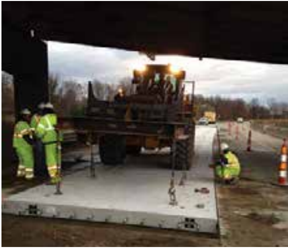
Figure 3-26. Placement of repair panels beneath an overpass on westbound Interstate 94 (Business Loop) near Kalamazoo, Mich.
