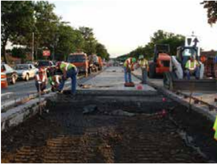
Figure 2-12. Undercutting foundation prior to placing PCP panels on Route 7 near Rotterdam, N.Y.
