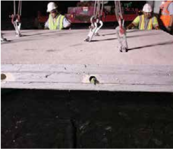
Figure 12-12. SwiftLift lifting inserts are favored by some precasters because they allow quick and safe attachment of lifting cables to precast panels.
