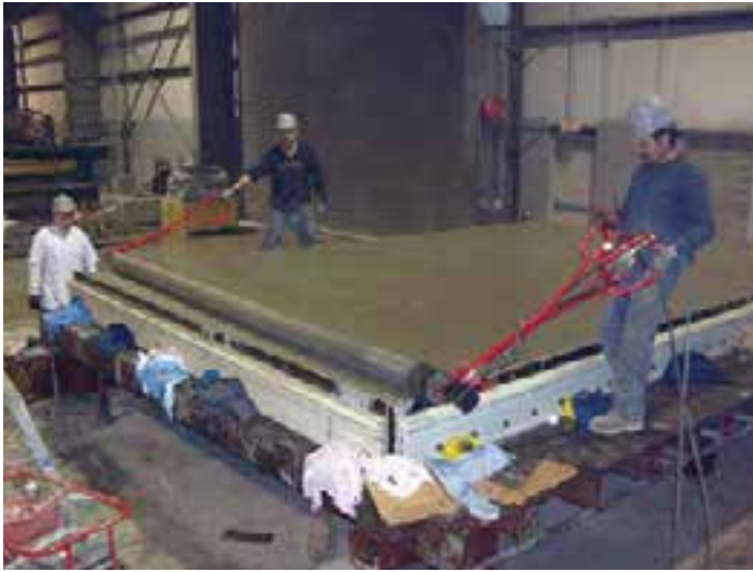
Figure 7-21. A hydraulically powered roller screed saves labor and time, producing a more accurate panel surface.
