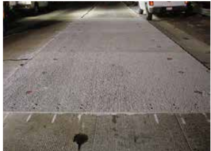
Figure 11-27. These panels, finished at the precast plant with a burlap drag-and-raked finish, did not require diamond grinding. Friction requirements were met during panel fabrication and smoothness requirements were met during panel placement.
