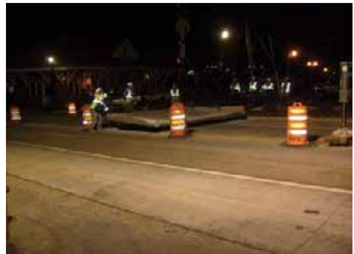
Figure 11-19. The damaged panel, less the concrete around the dowels, is removed.
