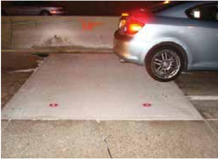
Figure 3-2. Eight-foot-long, full lane-width joint repair panel placed in a single lane.
