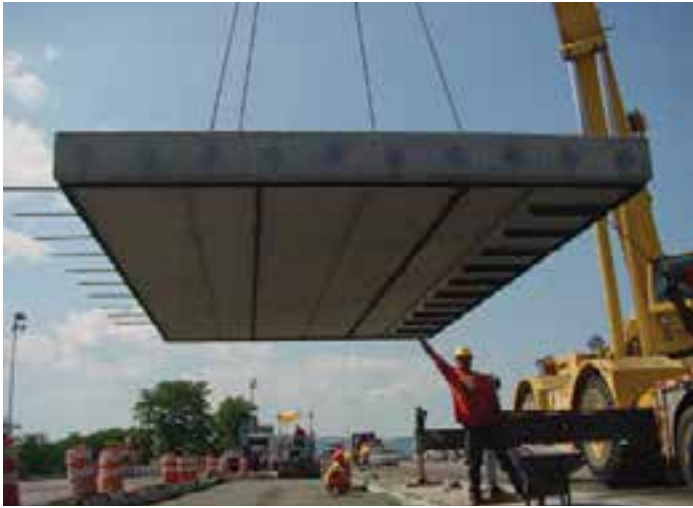
Figure 9-17. The bottom of a Super-Slab panel with built-in bedding grout distribution channels and black grout retention gaskets.
