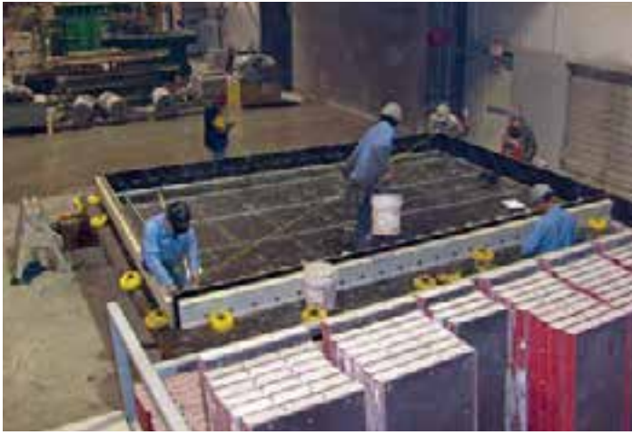
Figure 7-14. Checking form diagonals during form setup.
