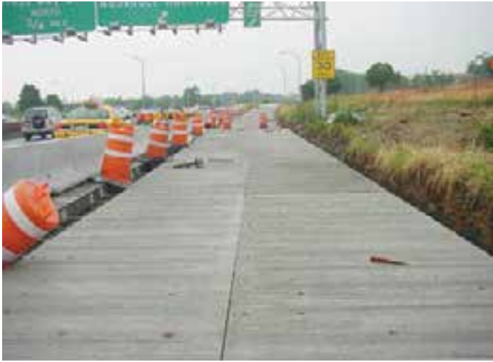
Figure 4-4. Wide precast concrete ramp pavement in Long Island, N.Y., with a longitudinal joint in the center of the lane.
