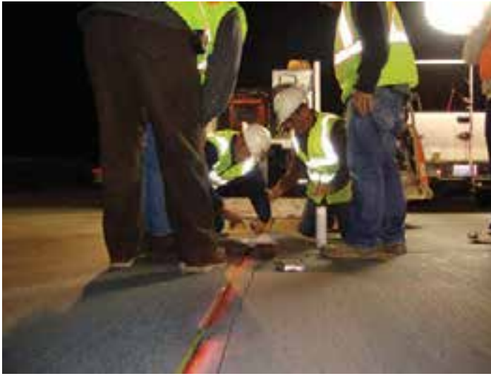
Figure 10-6. A contractor's crew checks saw cut layout lines prior to sawing.
