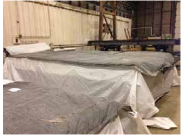
Figure 7-25. A newly casted panel covered with plastic and insulating blankets for initial curing.
