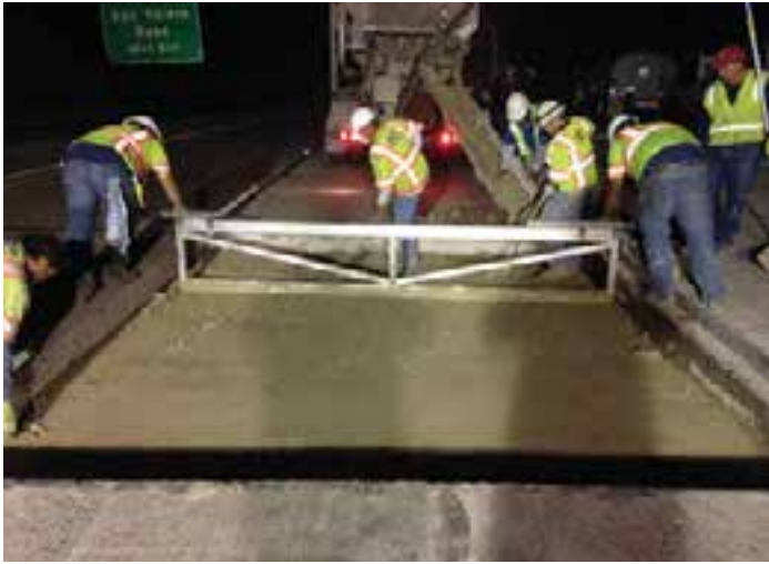
Figure 9-7. A wheel-mounted concrete screed using a pre-set rail on one side of the hole and the existing pavement on the other as a grade reference.
