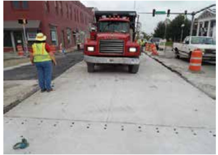
Figure 4-5. Installation of wide panels (travel lane plus shoulder) in Winder, Ga.
