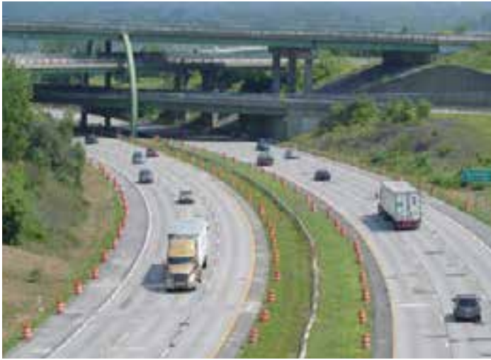
Figure 3-4. Use of precast panels for joint and mid-slab crack repairs in 62-foot-long slabs.
