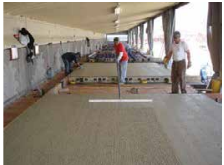
Figure 7-23. Commercially available rake being used to impart macrotexture on top of a previously applied burlap drag ("microtexture") finish.
