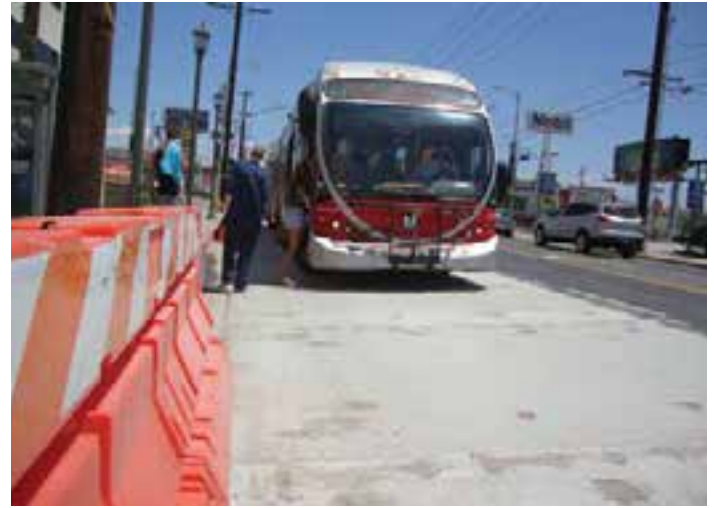
Figure 3-25. New precast bus pad pavement in North Hollywood, Calif.
