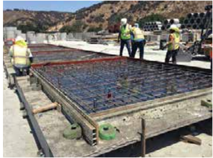
Figure 7-9. Aluminum extrusions (faced with special plywood) anchored with magnets in a long-line bed.
