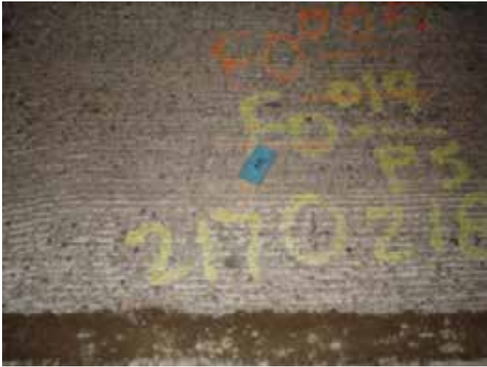
Figure 8-12. Example leading end mark for a panel designated number 217 (see black line perpendicular to pavement edge in yellow circle).
