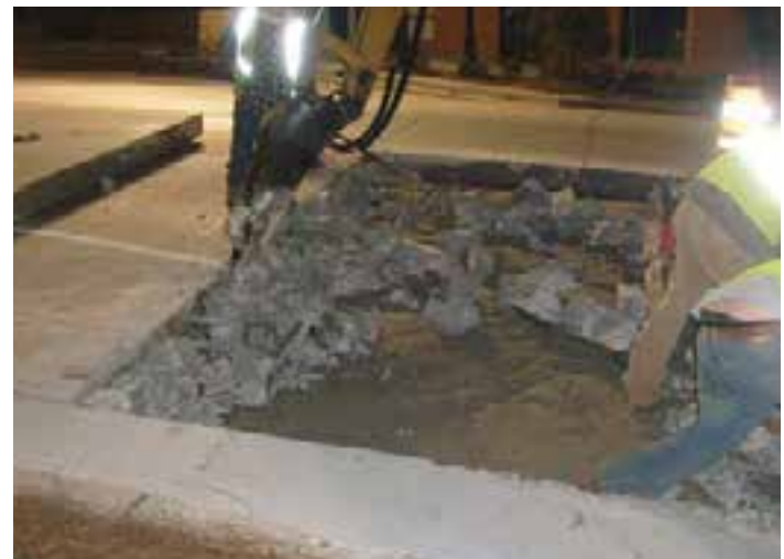
Figure 11-20. A small hoe ram removing concrete around dowels that are to remain in place.
