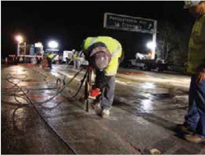
Figure 8-20. A concrete chainsaw equipped with diamond teeth is used to finish a full-depth saw cut without overcutting into the adjacent panel.
