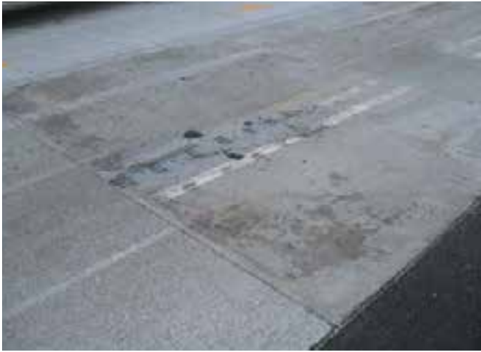
Figure 11-23. Non-uniform surface texture resulting from partial coverage by diamond grinding machine.
