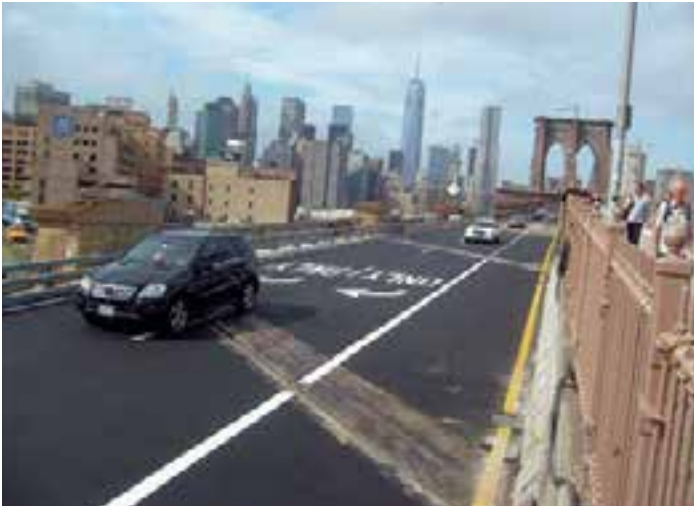
Figure 3-19. Only the header portions of the skewed precast approach slab panels used on this Brooklyn Bridge project in New York City are visible in this photo. All other precast panel exposures were overlaid with asphalt to provide a smoother riding surface.
