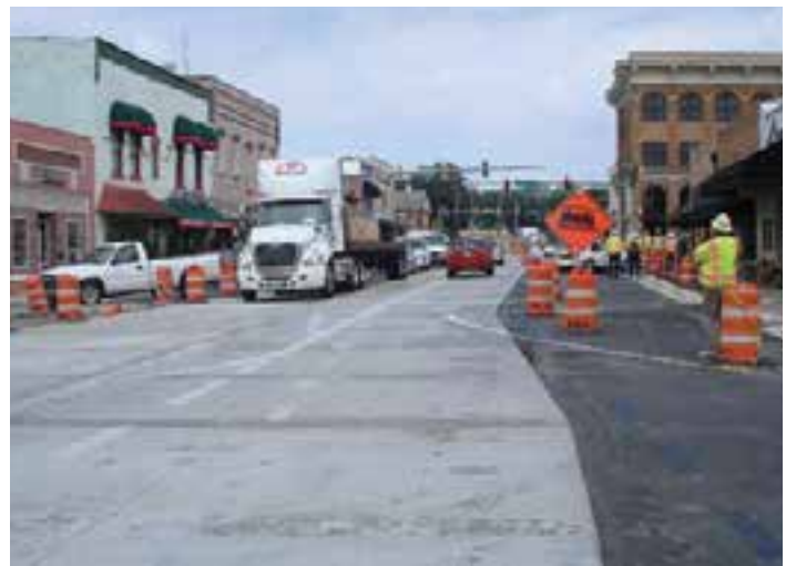
Figure 3-18. New precast panels on Broad Street in Winder, Ga.
