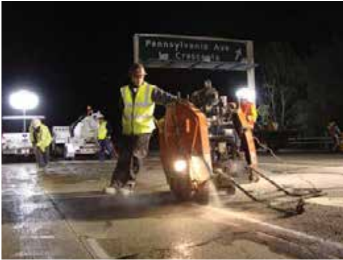
Figure 8-17. This sawing crew is equipped with adequately sized saws, proper lighting, a water supply and a slurry suction truck.
