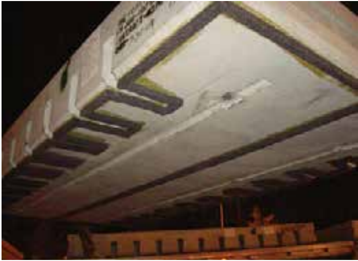
Figure 4-10. Proprietary grout distribution channels and gasket material on a Super-Slab JPrCP panel.
