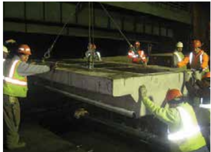
Figure 3-29. Weigh-in-motion precast unit being lowered into position in the field.
