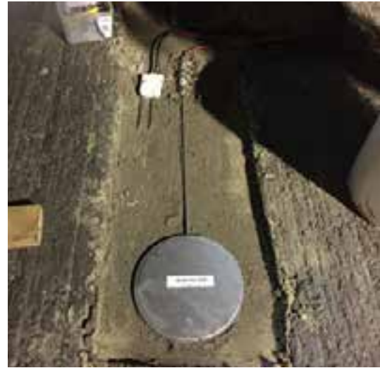
Figure 13-16. A moisture sensor and load cell being installed.
