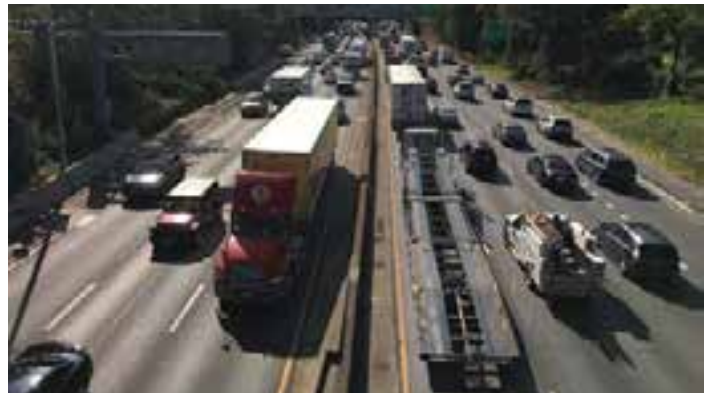
Figure 2-1. Example of a heavily trafficked route that may be subject to short repair work windows.
