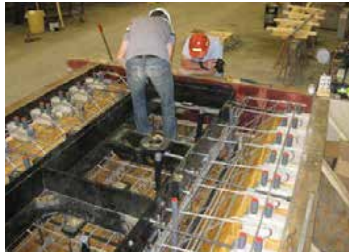
Figure 3-28. Frame for weigh-in-motion scales positioned in a precasting form.
