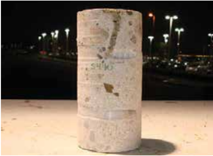
Figure 11-9. The shallow crack in this core, measuring approximately .02 inches wide at the top of the panel, stopped at the top layer of reinforcing.
