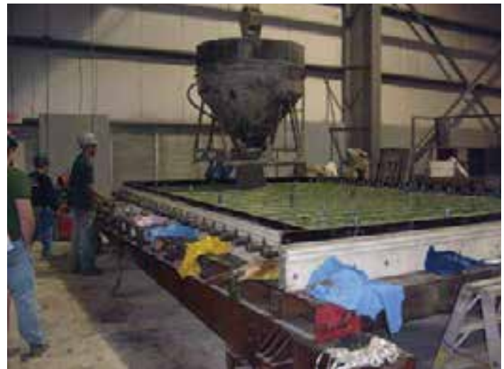
Figure 7-19. Use of a conventional concrete bucket to place panel concrete in a “high” form.
