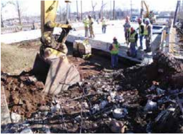
Figure 3-22. Replacement of bridge embankment material below approach slabs on the Route 46 Bridge in Clifton, N.J.
