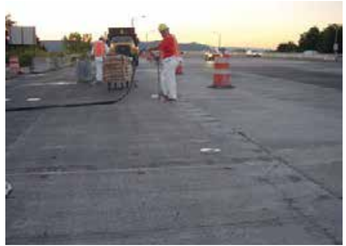
Figure 9-18. A worker pumping bedding grout into one end of a distribution channel until it comes out the other, a technique that verifies bedding grout has flowed under pressure for the entire length of the channel, indicating full distribution of grout under the panel.
