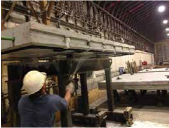
Figure 7-29. Application of sprayed curing compound to all panel surfaces.
