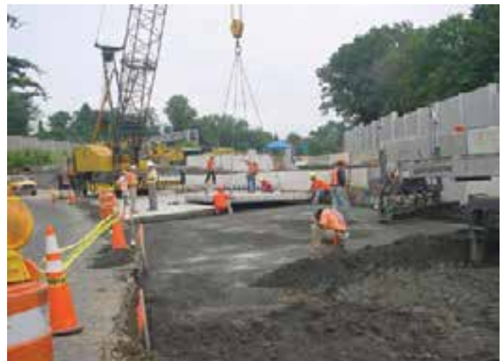
Figure 9-49 Because equal-length picking cables were used over a sloped surface, PCP panels on this project had to be placed numerous times to bring joint widths within specified tolerances.
