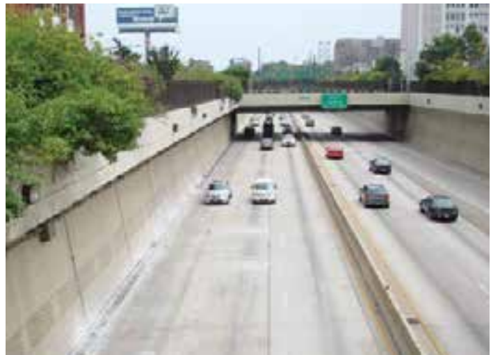
Figure 3-13. Intermittent precast repairs on Interstate 680 in Philadelphia, Pa.
