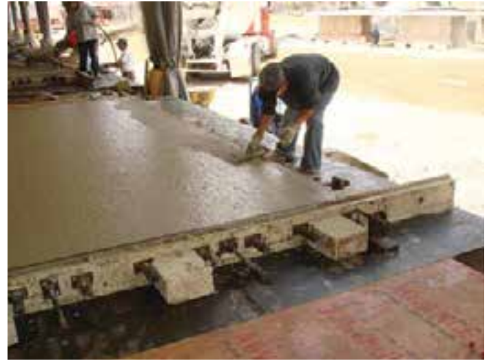
Figure 7-22. Worker touching up the screeded surface near the side rails.
