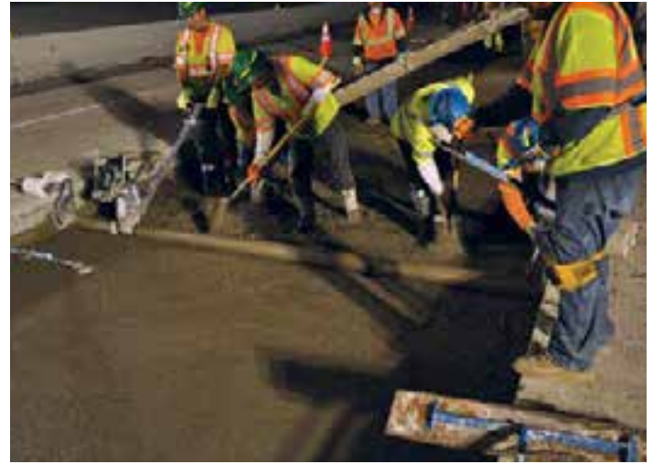
Figure 9-8. A "homemade" mechanized roller screed is used to screed new lean concrete base while masons hand-finish the new lean base on each side of the placement.
