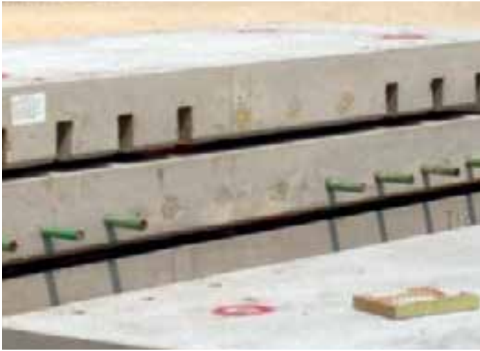
Figure 4-23. Precast panels with dowels translated vertically downward to provide thicker concrete over slots.
