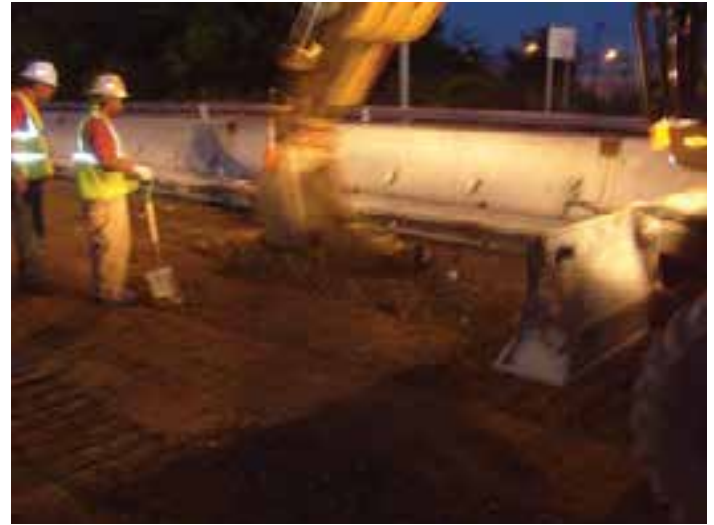
Figure 8-29. Spot repair during subbase preparation.
