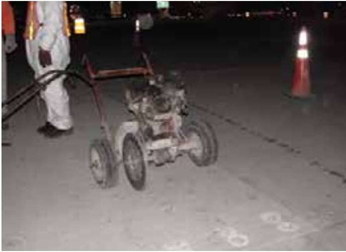
Figure 11-33. A joint cutting saw equipped with a stack of blades equal to the desired joint width.
