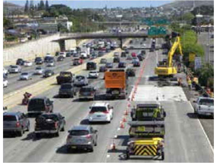
Figure 1-2. Precast pavement repair underway on heavily trafficked Interstate H1 in Hawaii.
