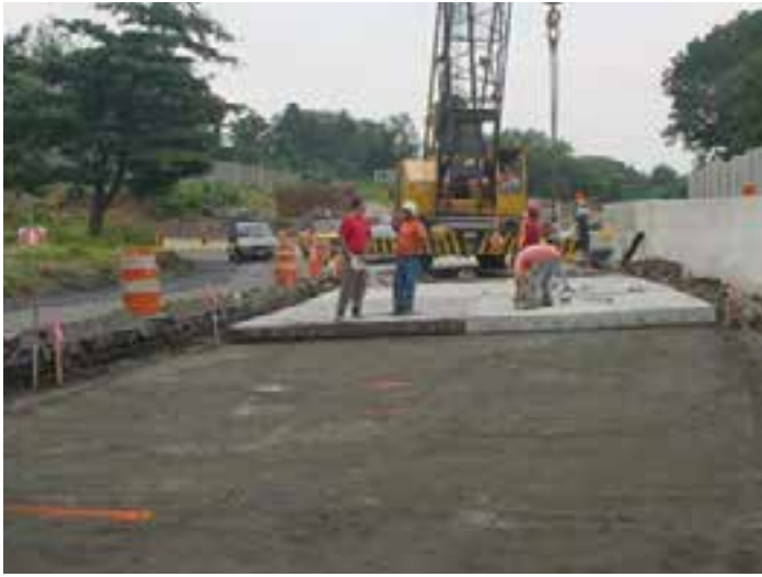
Figure 8-15. Panel points, identified with red paint, being used on a PCP project.
