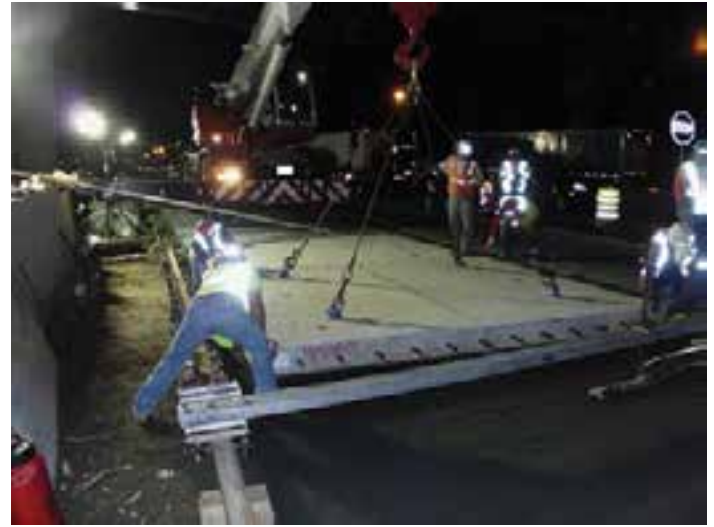
Figure 2-3. Example installation of PCP in a single-lane closure.
