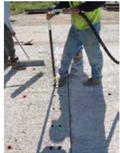
Figure 9-27. Injection of structural grout in dowel grout ports. Momentary pressure – to ensure the bottom slot is completely filled – is developed when an installer places a foot over the front port while dowel grout is pumped into the back port.
