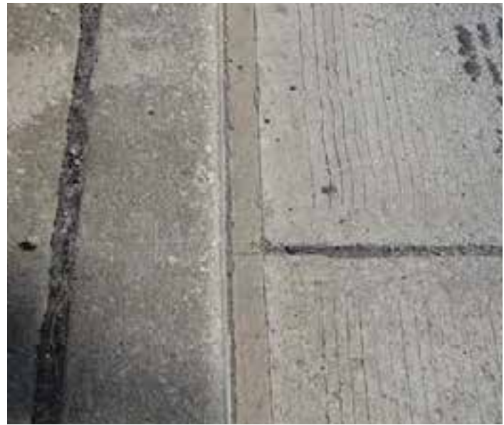
Figure 12-7. This 1.5-inch-wide, grout-filled longitudinal joint, located between an existing curb on the left and precast panels on the right, is performing well after being in service for more than five years.
