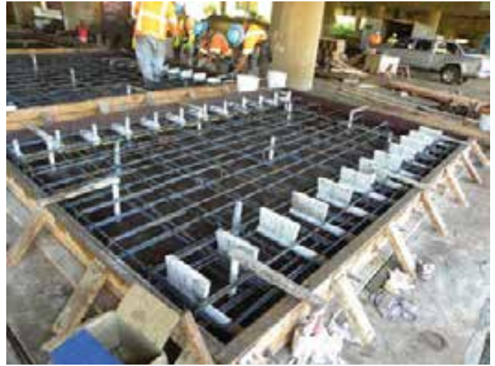
Figure 7-5. Plywood forms used at a contractor's on-site "precast yard" under an overpass.
