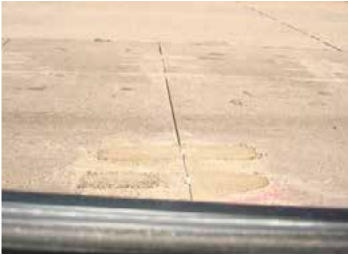
Figure 11-5. The original dowels in the top slots seen in the foreground were sawed out and replaced with new, full-length dowels and the slot was backfilled with polyester concrete.
