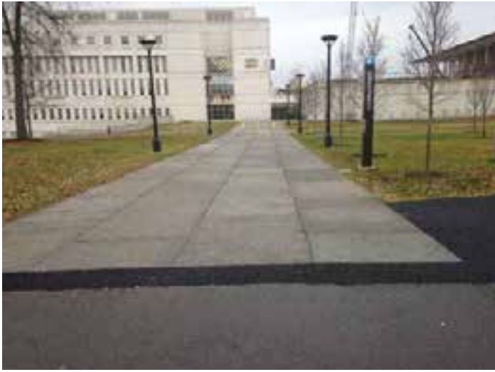
Figure 13-18. The sidewalk in this photo consists of pervious precast panels.
