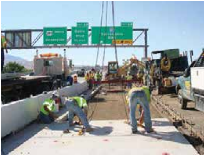
Figure 8-4. The work area allowed on this three-lane interstate was restricted to one lane, a small portion of the adjacent lane and the shoulder on the right.
