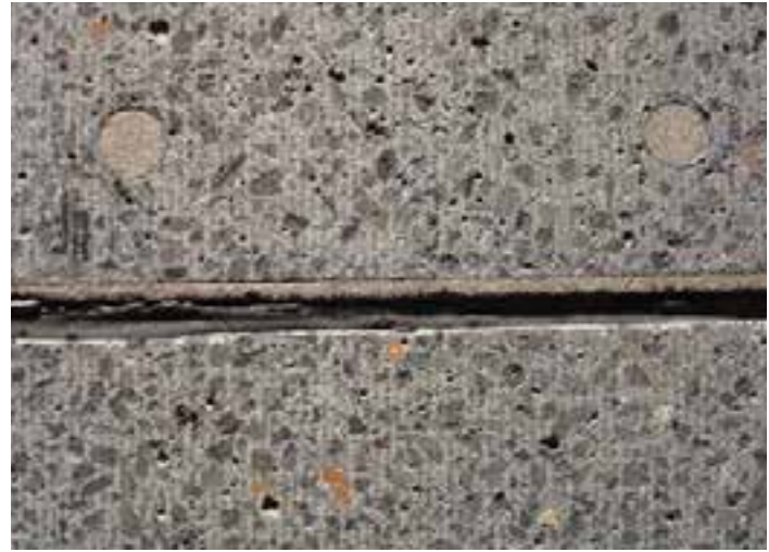
Figure 11-34. The sealant reservoir in this over-width joint was incorrectly cut with a 1/2-inch-wide blade. The remaining grout has already de-bonded from the existing pavement and is ready to fall out of the joint.
