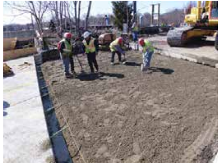
Figure 10-15. A grading crew using string lines (foreground) to check the rough grade of bedding material.
