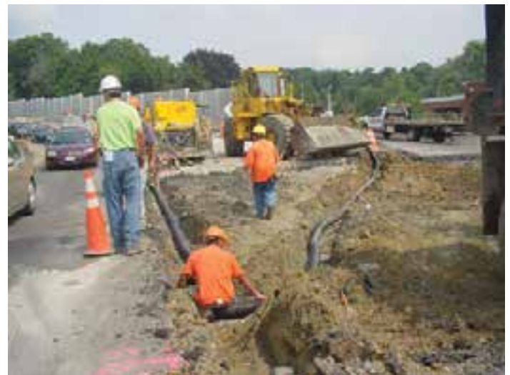
Figure 8-30. Extensive subbase repair prior to JPrCP installation (visible in the background).
