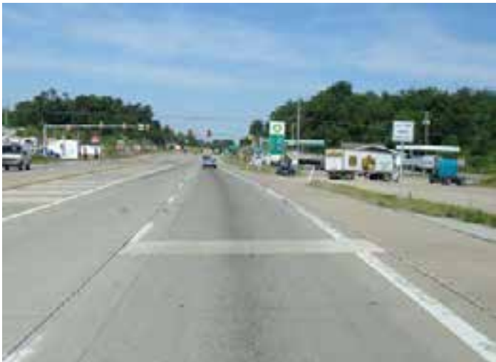
Figure 4-3. Concrete pavement with widened outside lane construction.
