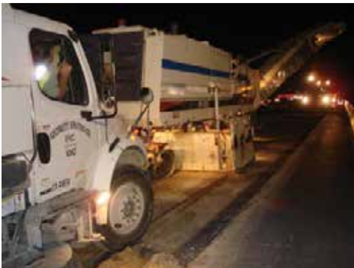
Figure 8-33. CTB removal with a large-scale milling machine, followed by a conventional "street sweeper" broom truck to ensure all milled material is removed.
