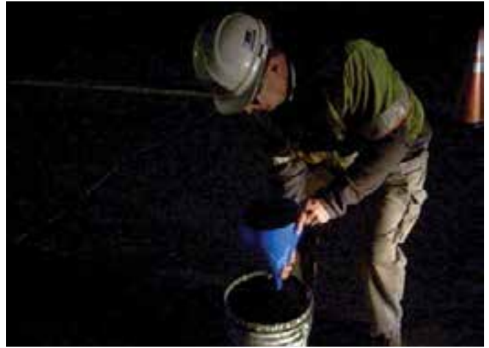
Figure 9-14. A worker performs a flow test in accordance with ASTM C939 to ensure proper consistency of the bedding grout.
