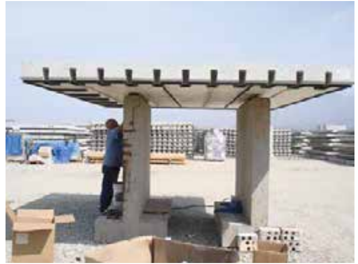
Figure 7-27. Applying foam gaskets to bottom of Super-Slab panels that have been placed on high stands.
