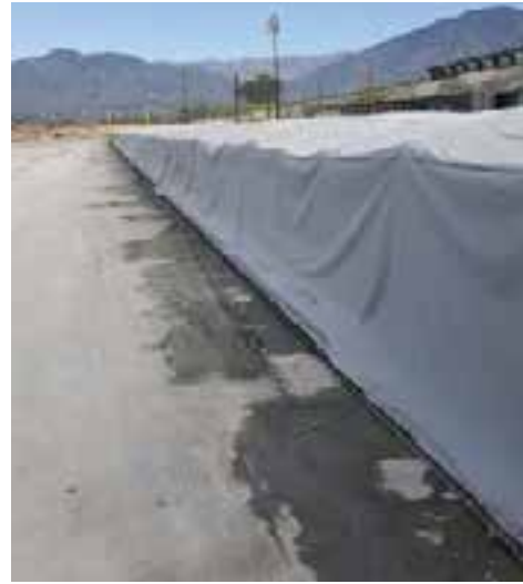
Figure 7-2. Long-line bed covered with insulated curing blankets to facilitate steam curing.
