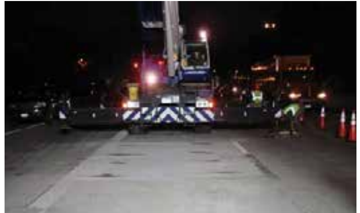
Figure 8-1. Men working approximately 8 feet away from live traffic, separated only by widely placed traffic cones.
