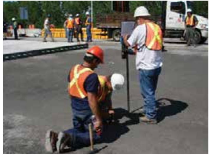
Figure 8-16. Survey crew using a robotically controlled total station to lay out panel points on a total replacement project.
