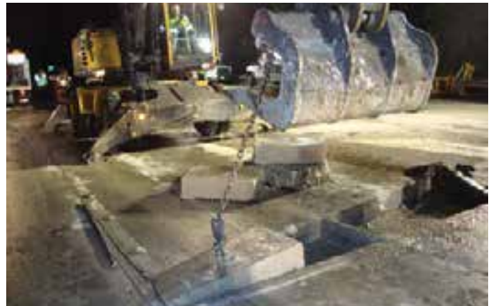
Figure 8-25. Excavator removal using a slab-crab bucket, showing little disturbance of the underlying subbase.
