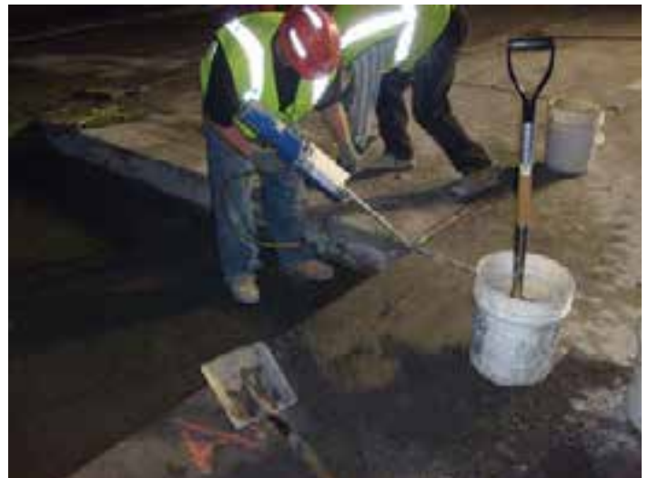
Figure 8-19. Filling a transverse overcut with dowel bar epoxy anchoring material.
