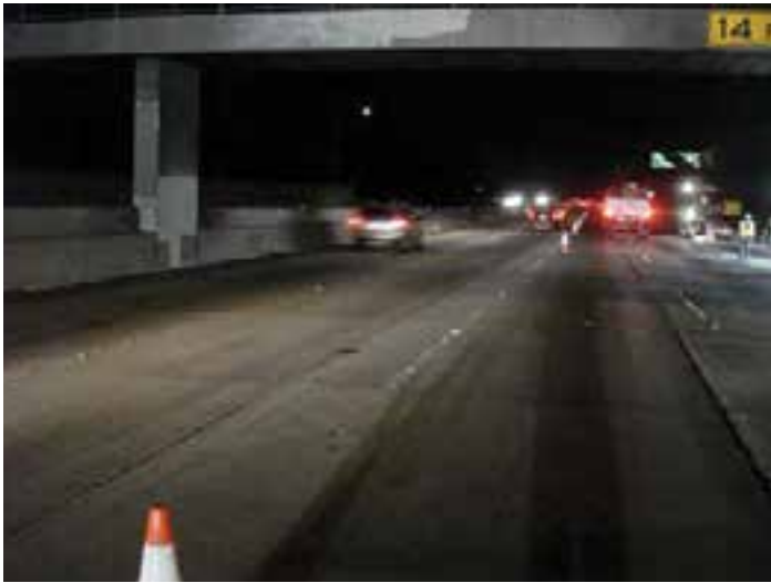
Figure 8-2. The work area on this five-lane California interstate project was three lanes wide, providing a safe, 12-foot-wide buffer zone.
