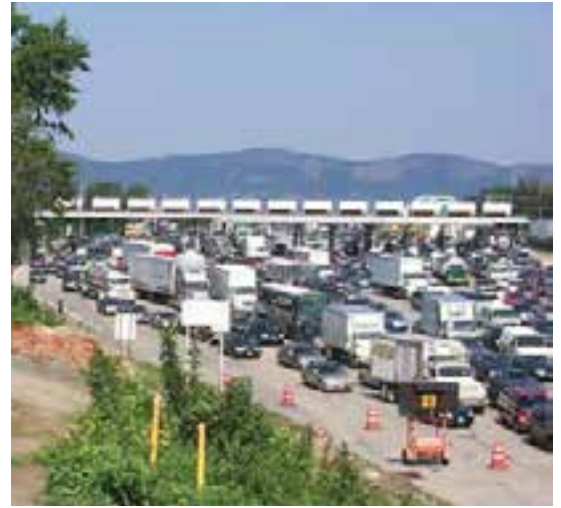
Figure 3-20. Rush hour traffic at the Tappan Zee Bridge toll plaza near Tarrytown, N.Y., in 2000 before the plaza was replaced with new JPrCP panels.
