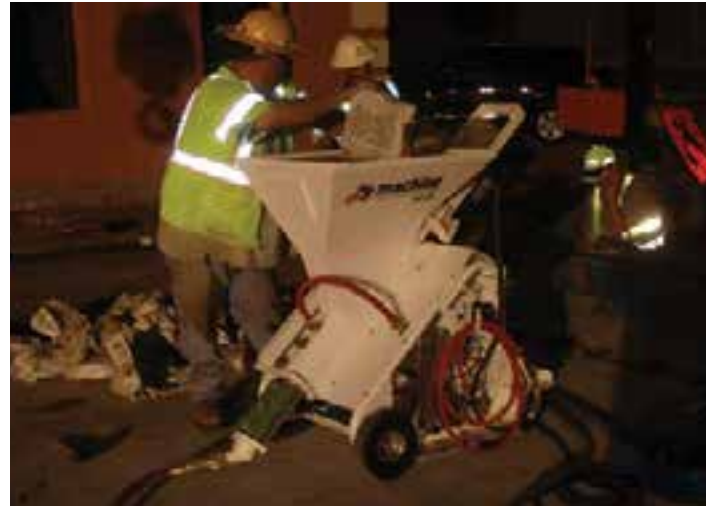
Figure 9-16. Workers dumping grout powder into the top of a volumetric mixer/pump.
