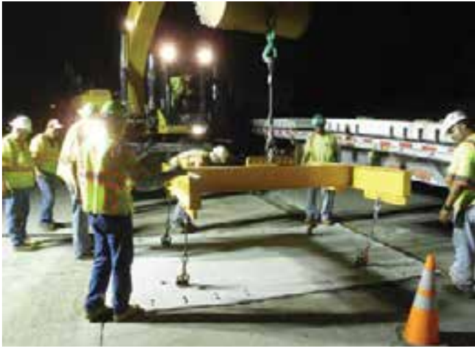
Figure 9-45. A rubber-tired excavator placing a 12-foot-wide-by-10-foot-long panel that was “picked” from the truck positioned alongside.
