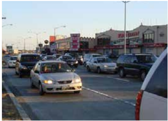
Figure 3-12. Precast concrete lane replacement on Rockaway Boulevard in Queens, N.Y.
