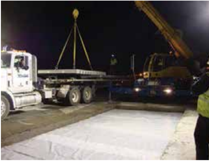
Figure 10-5. Panels arriving on trucks are easy to inspect for defects and flaws because all six surfaces of each panel are visible.
