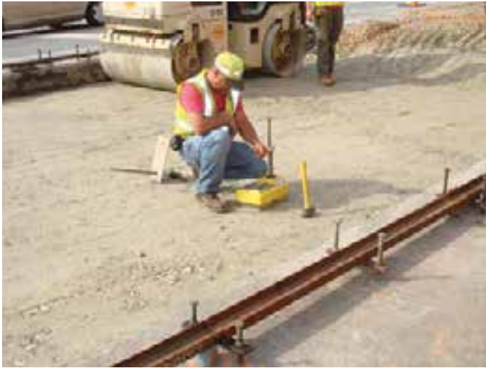
Figure 8-28. Density testing of newly placed subbase material to evaluate compaction.
