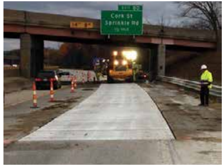
Figure 8-5. Traffic being diverted to the left shoulder, leaving a partial lane, a full lane and the shoulder on the right as a safe working area.
