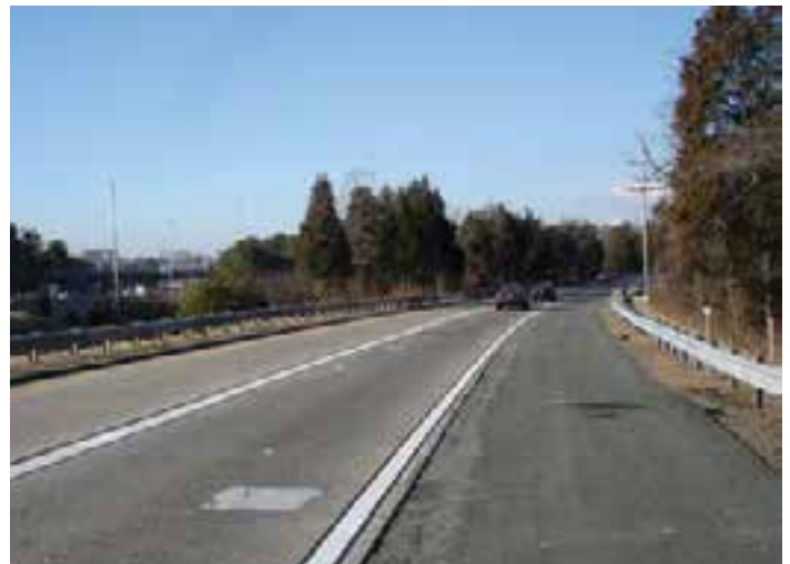
Figure 3-11. The right-hand lane of a high-speed exit ramp in Fairfax, Va., that was replaced during overnight full ramp closures.
