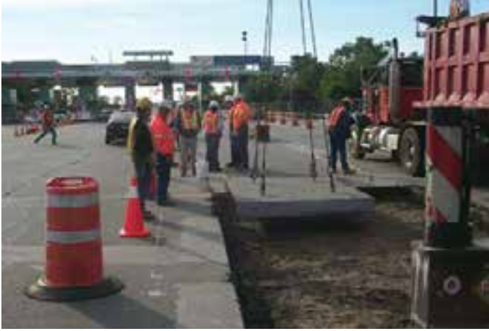
Figure 8-22. Slabs being removed using the lift-out method. Notice the spalls on the edge of the remaining pavement on the left caused by the lifting operation.
