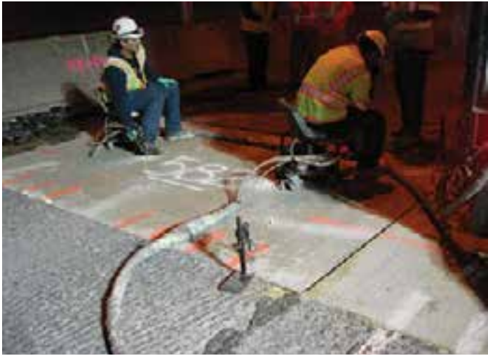
Figure 9-11. Two workers, each equipped with a urethane injector tip, installing foam to the underside of the panels through foam ports.
