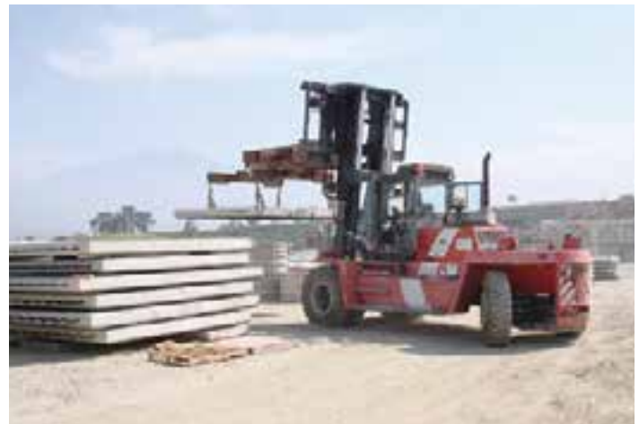
Figure 7-31. Moving, stacking and storage of precast concrete panels.
