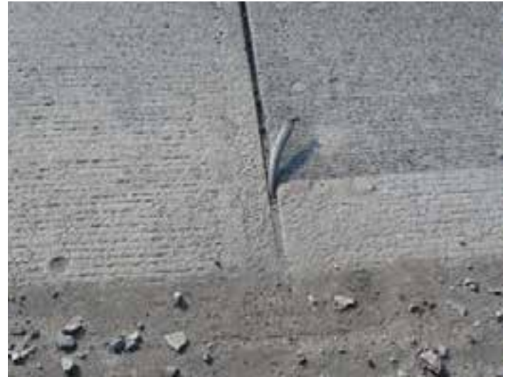
Figure 12-9. The bond between the silicone seal and concrete failed after approximately five years of service in this constant-width joint. Joint cleanliness problems during installation are suspected.
