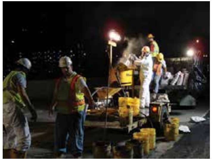
Figure 10-18. On-the-job training of a grout crew.
