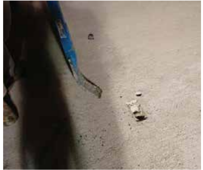
Figure 12-13. Recesses required for SwiftLift lifting inserts are elliptical in shape, providing little resistance to grout pop-out.
