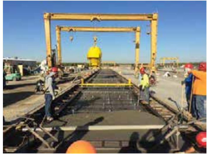
Figure 7-4. Long-line prestressing beds with adjustable end rails.
