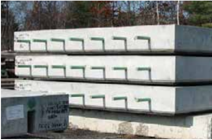
Figure 4-16. Half-embedded dowels in a JPrCP panel.
