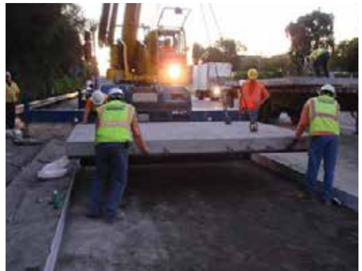
Figure 10-16. An ideally sized panel placement crew of five, with one man in each corner and one man on the truck.
