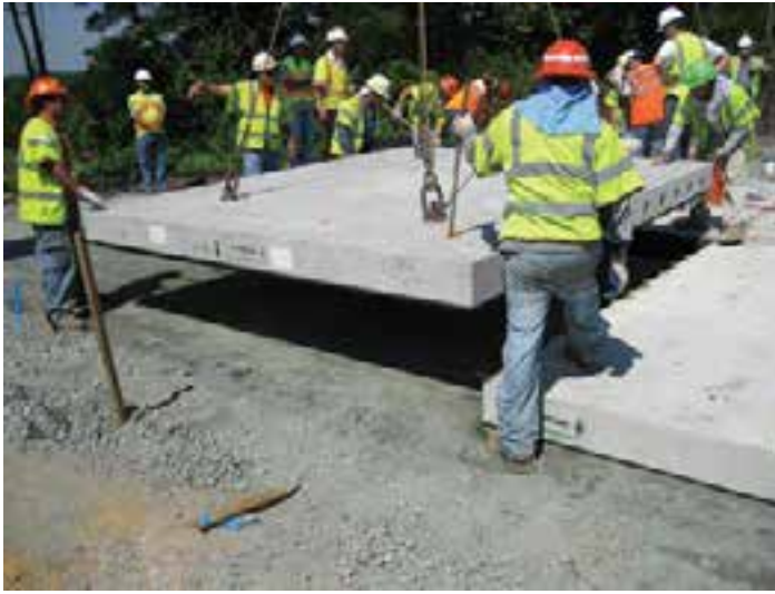
Figure 10-1. State DOT engineers witness the installation of a precast panel at a system trial installation.
