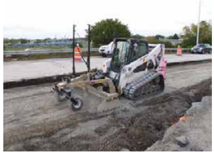
Figure 9-4. A laser-equipped skid-steer and grading box using a digital surface model for grade control.
