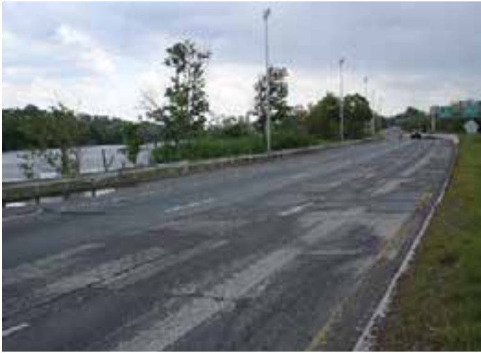
Figure 3-30. Milled composite pavement on Route 21 in New Jersey.
