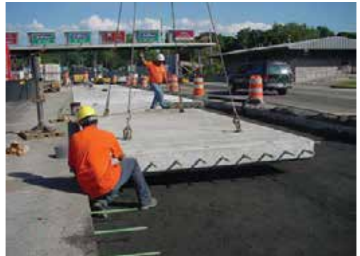
Figure 4-9. Placement of grade-supported precast panel for overnight use prior to installation of bedding grout at Tappan Zee Toll Plaza in New York.
