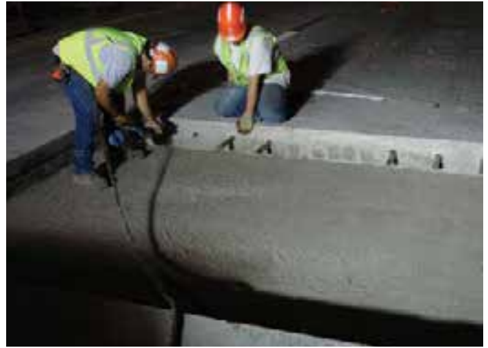
Figure 9-26. An air-powered, epoxy injection (caulking) gun is used to install anchoring epoxy. White epoxy retainer discs are visible around the dowels.
