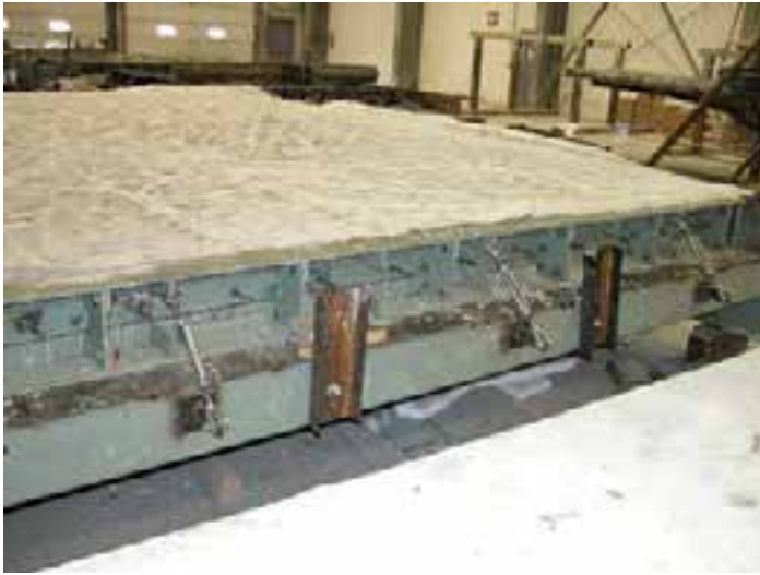
Figure 7-8. Turn buckles and push bolts are used to keep the tops of side rails straight.
