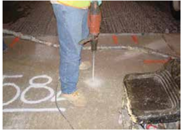
Figure 9-12. A worker drills a new foam port in a part of the panel that needs extra force to provide vertical uplift.
