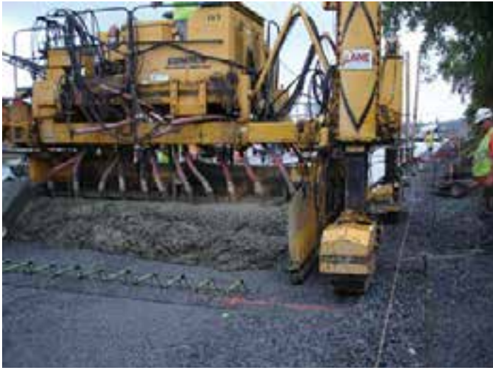
Figure 1-3. String line controlled slip-form paver approaching dowel basket (note vibrators for consolidation).
