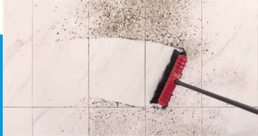
Wet Sweep – spray a water mist to keep dust down while sweeping
