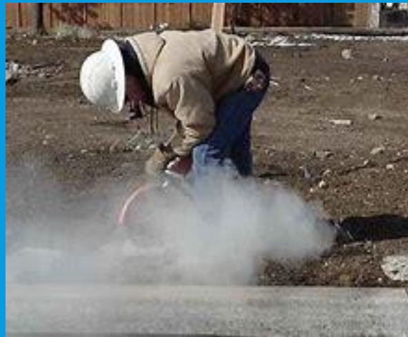
Concrete saw dust
