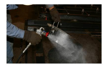
Spray systems can put form oil into the air. The PELs for PNOR and respirable vegetable oils are 5 mg/m<sup>3</sup> (milligram per cubic meter).
