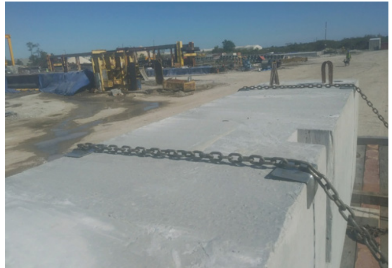
Correct strapping with chain guards
