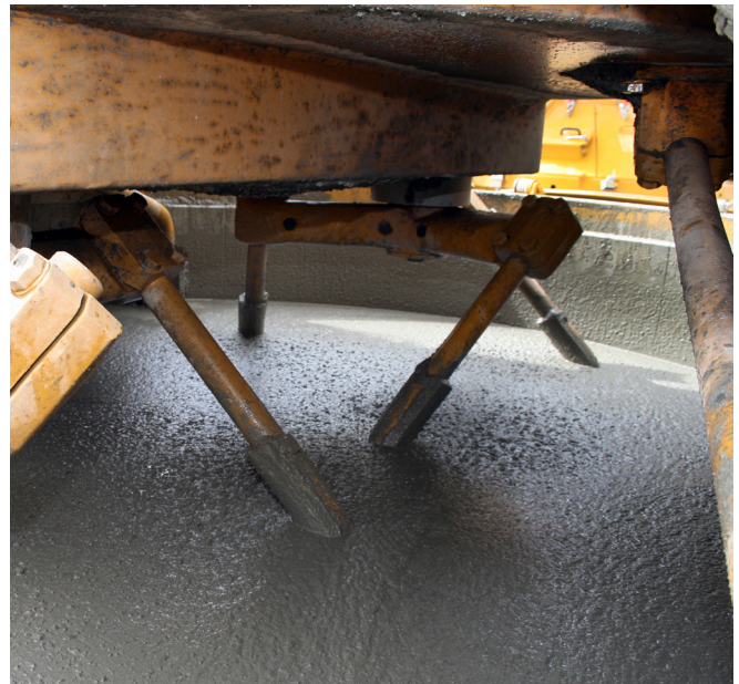
High-Range Water-Reducers are efficient in producing self-consolidating concrete.
