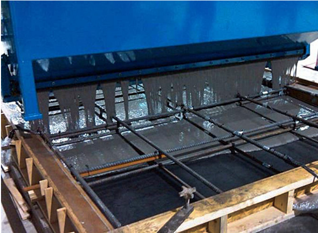
Figure 4 – Placing UHPC behind the leading edge. (Photo courtesy of Lafarge)
