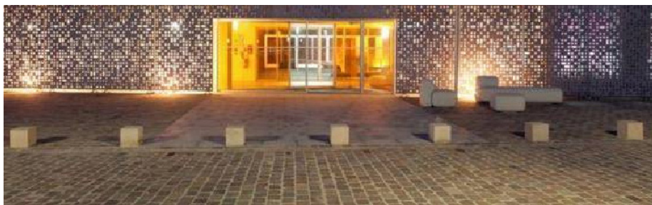
Figures 15, 16 – Community Center, Sedan, France — perforated UHPC panels create a double-skin facade that provides privacy, sunshade and daylight.
