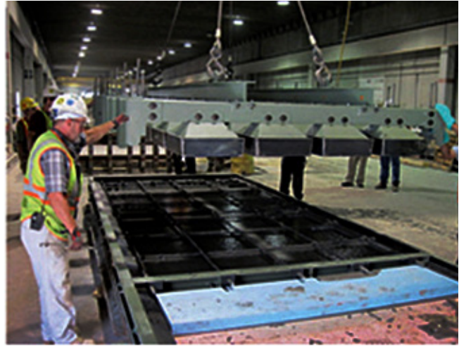
Figure 7 – Displacement casting. (Photo courtesy of Lafarge)
