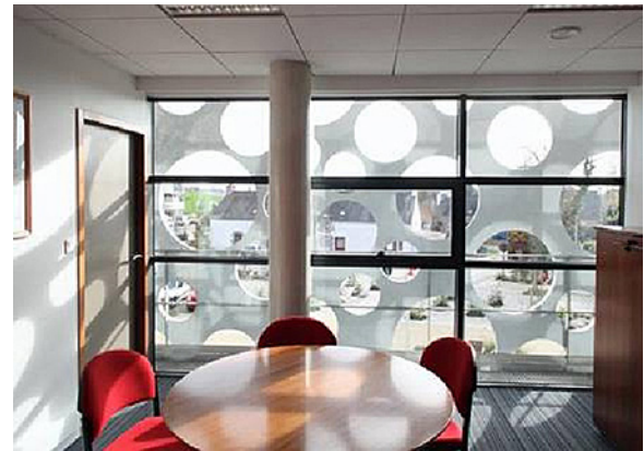
Figure 17 (top, left) – Lattice panels being formed with a vacuum injection molding system. Figures 18, 19: Perforated UHPC panels at Plescop City Hall, France. (Photos courtesy of Lafarge)
