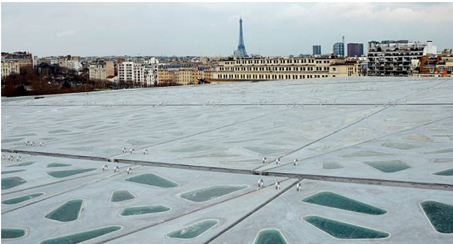
Figure 33 (left) – Stade Jean Bouin’s UHPC lattice roof system with glass inserts. (Photo courtesy of Olivier Amsellem). At right, the open lattice facade allows sunlight to filter through. (Photo © courtesy of Lisa Ricciotti).
