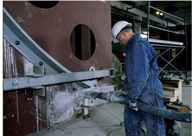
Figure 5 – Injection casting. (Photo courtesy of Lafarge)
