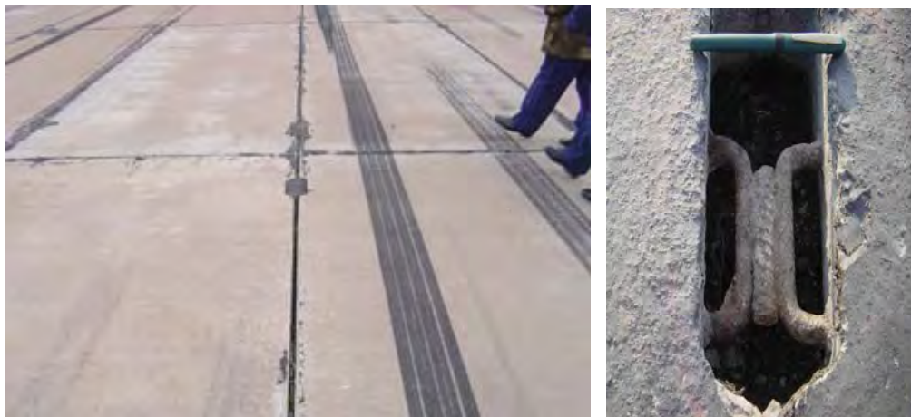
Figure 2.15. Soviet-era precast panels.
