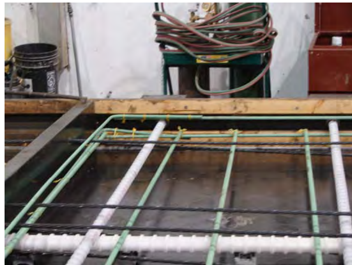
Figure 9.4. Prestressing steel-related hardware.
