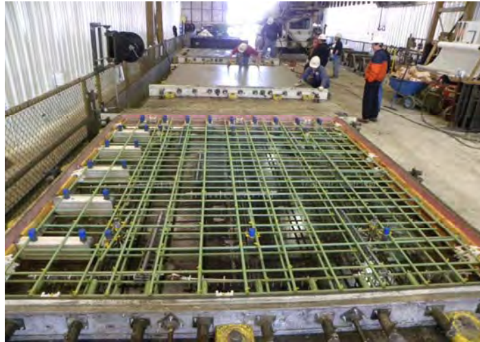
Figure 9.3. Reinforcement placed in both directions. (Courtesy of FMC)
