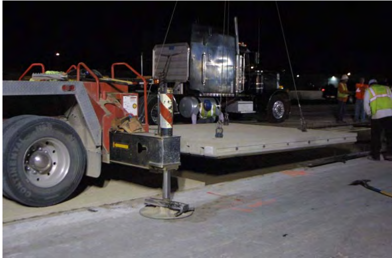
Figure 4.4. Outrigger positioning of lifting crane.
