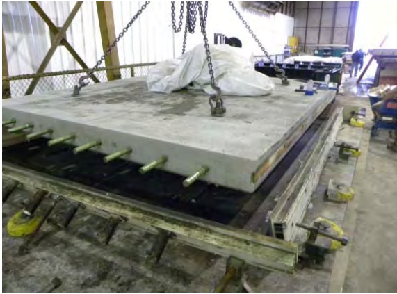
Figure 4.2. Typical four-point lifting of a precast panel.
