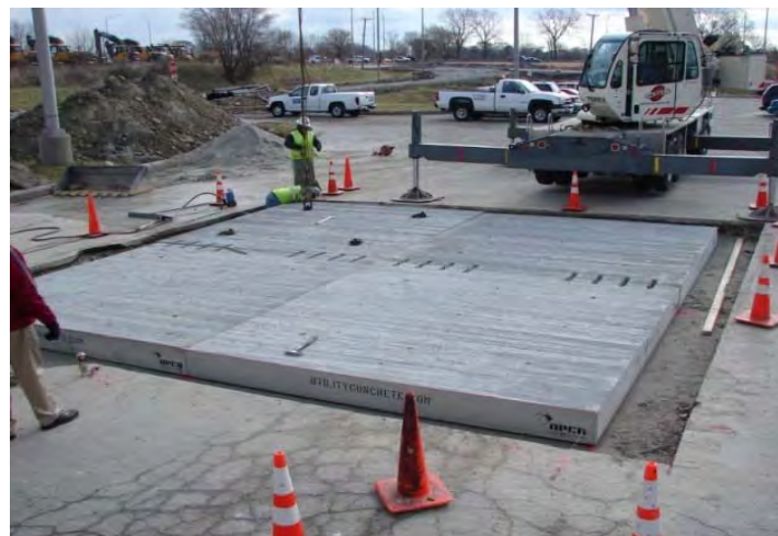
Figure 2.13. Illinois Tollway intermittent repair system.
