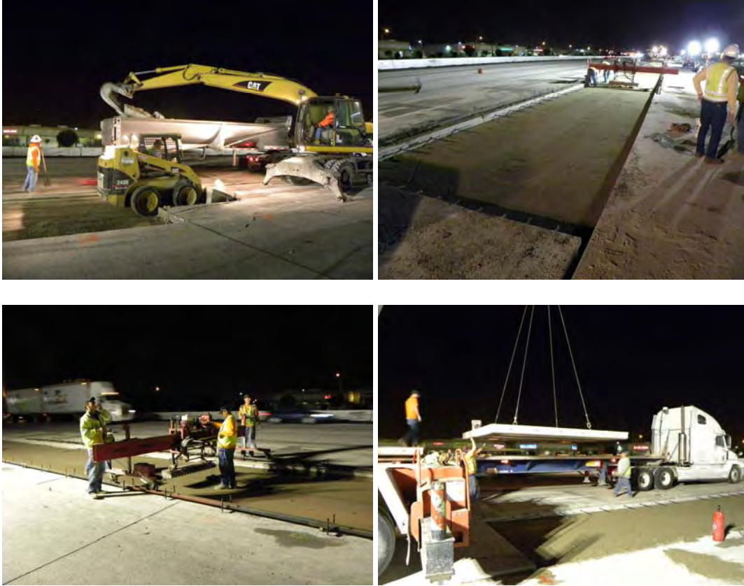
Figure 15.3. Lane closure scenario for a continuous PCP application.
