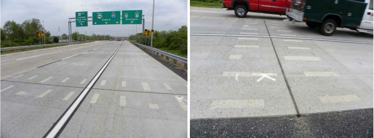
Figure 3.21. Views of the Delaware PPCP project.
