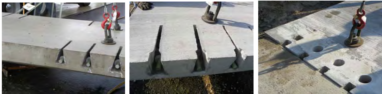
Figure 14.8. Three versions of the sliding dowel bar technique
