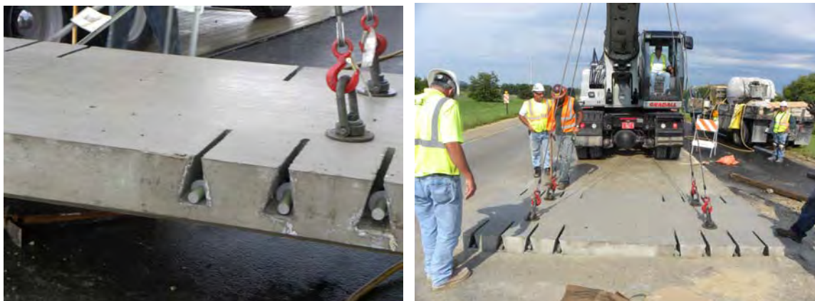
Figure 14.5. Narrow-mouth surface dowel slots.
