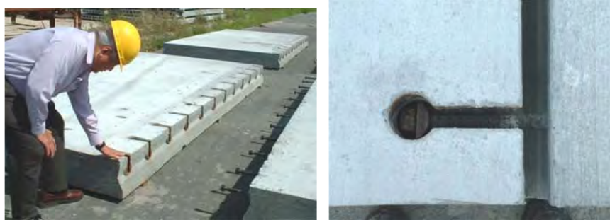
Figure 2.12. The Kwik Slab joint interlocking system.
