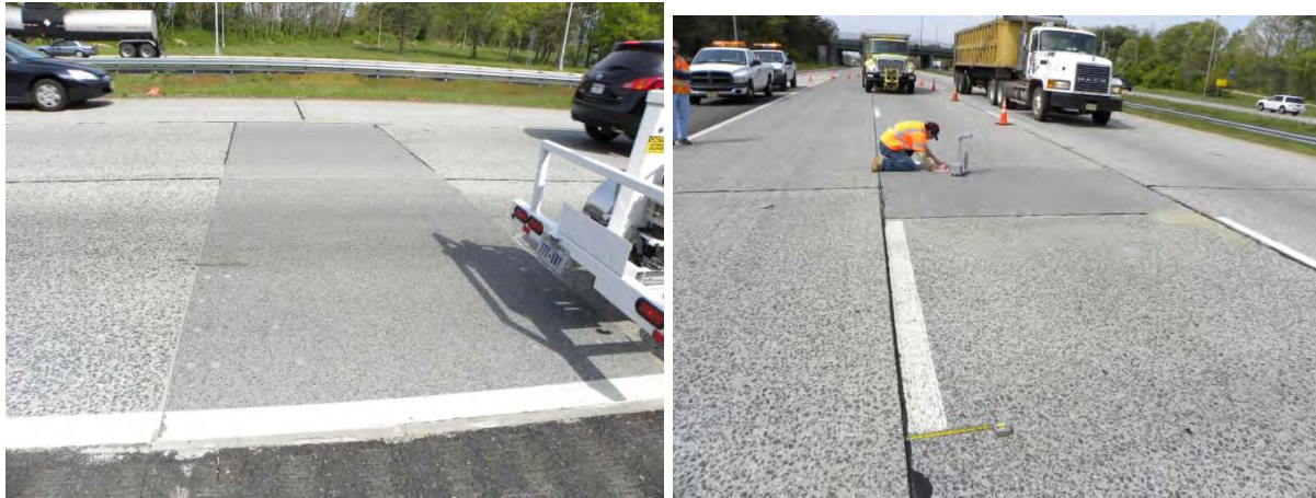
Figure 3.3. Views of the I-295 precast panels.
