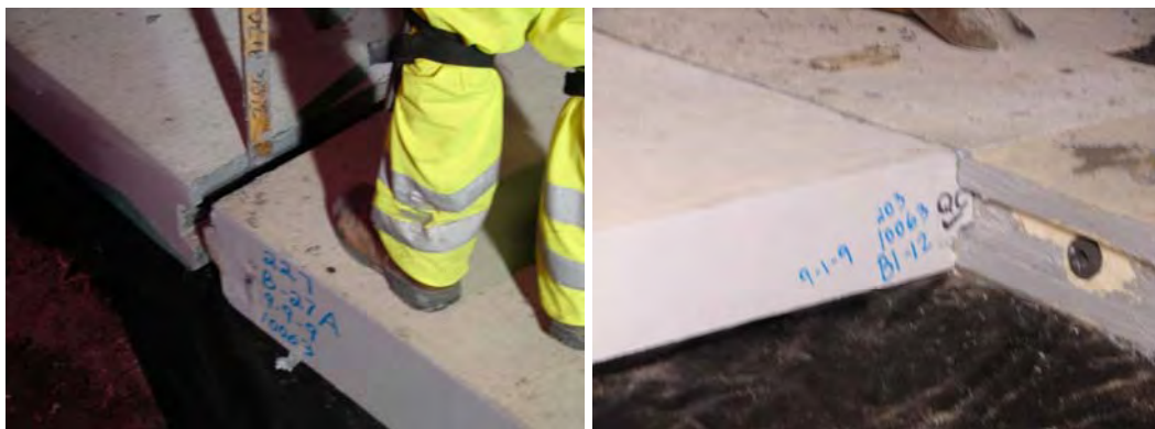
Figure 12.5. Intermediate keyway joint.
