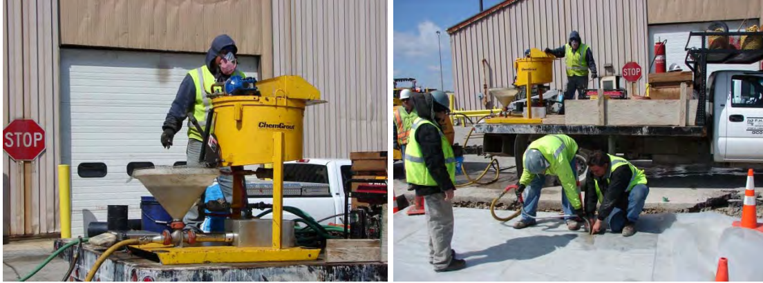
Figure 10.9. Undersealing grout pump and grouting operation.
