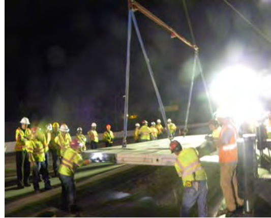
Figure 4.2. Typical four-point lifting of a precast panel.
