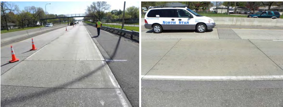
Figure 3.9. Views from the Minnesota project (precast panels in right-hand lane).
