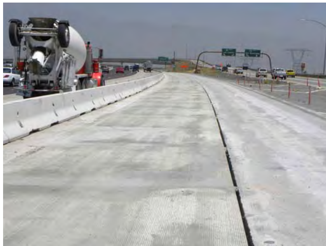
Figure 3.12. View of the I-15 JPrCP project.
