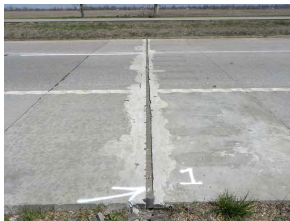
Figure 3.18. I-57 PPCP-reconstructed expansion joint.
