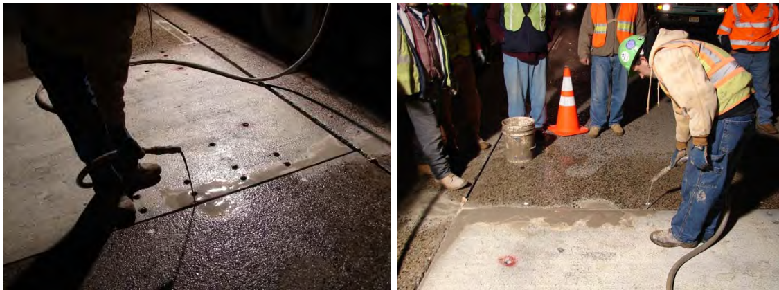
Figure 10.7. Dowel slot grouting.
