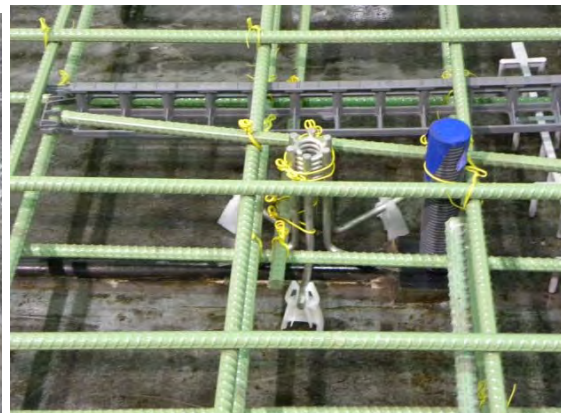
Figure 4.3. Lifting anchors. (By permission of FMC)
