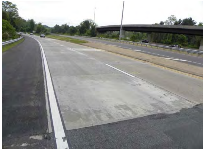
Figure 3.10. View of the I-66 JPrCP project.
