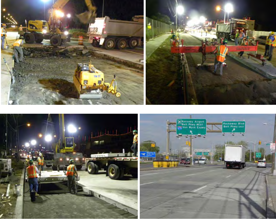
Figure 15.1. Completed installation at an intersection along Rockaway Boulevard.
