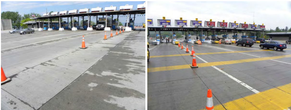
Figure 3.8. Approach and leave views of the Tappan Zee toll plaza.
