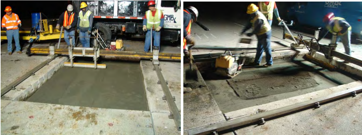
Figure 10.2. Base being graded and compacted within the repair area.
