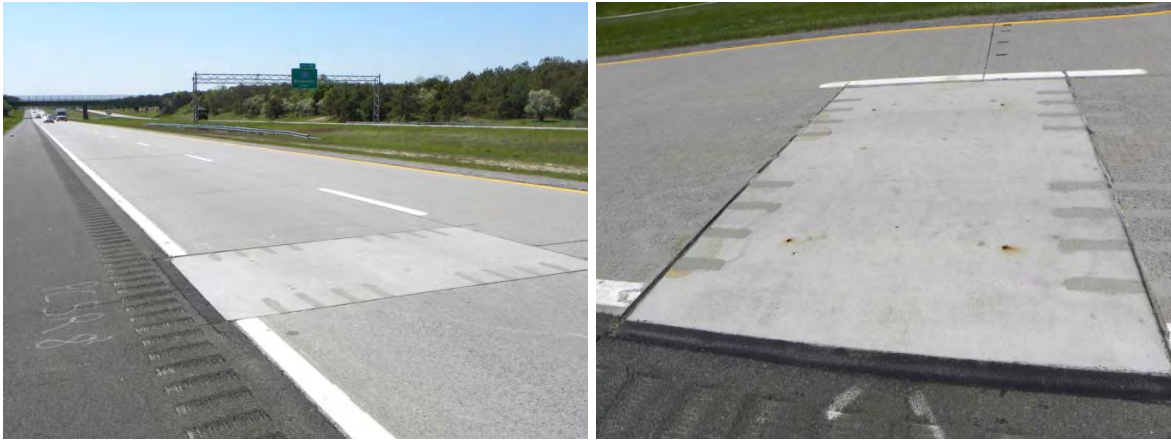
Figure 3.5. Views of the precast panels at the Route 27 project.
