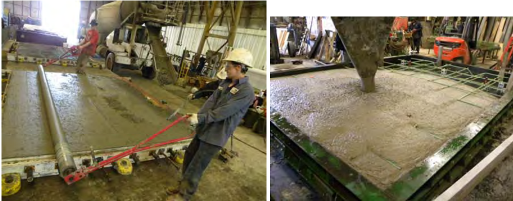
Figure 9.7. Two concrete placement processes (slump concrete and SCC).
