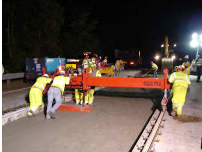
Figure 6.1. Auger-based granular base grading system.
