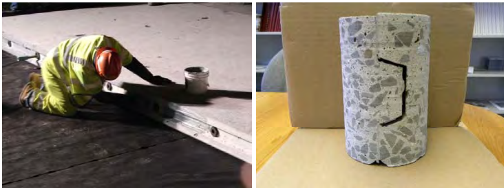
Figure 12.3. Applying epoxy along the transverse keyway joint face.
