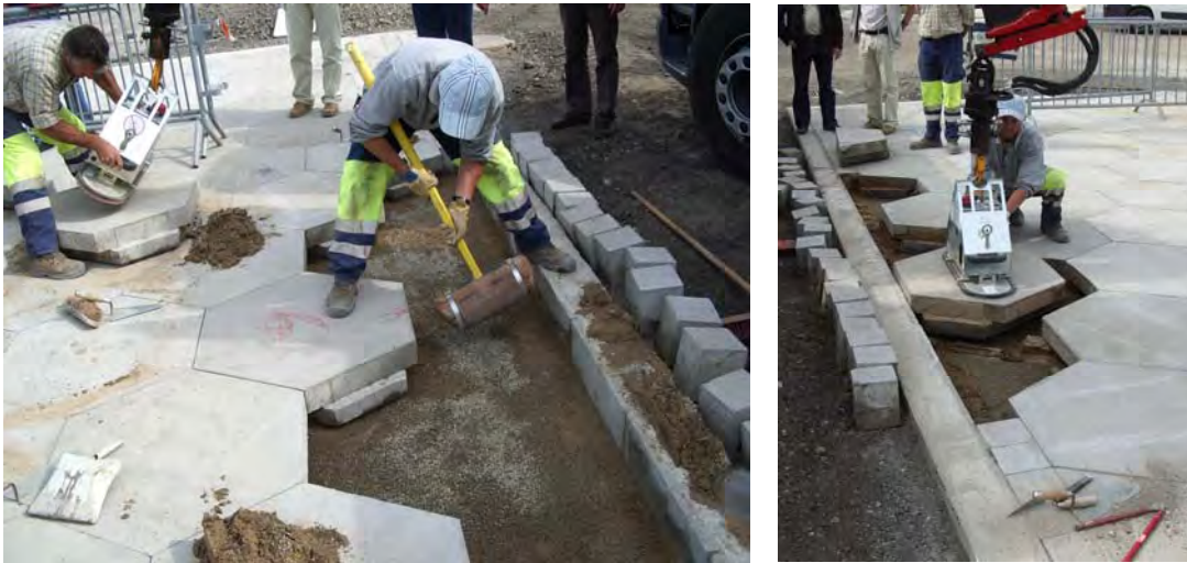
Figure 2.17. Installation of the keyed hexagonal panels.
