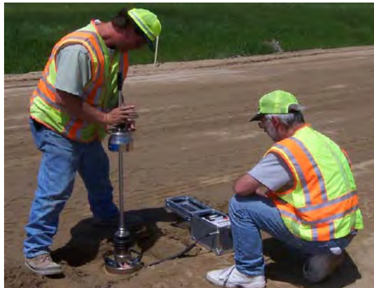
Figure 6.4. Light-weight deflectometer. (Courtesy: Minnesota DOT)
