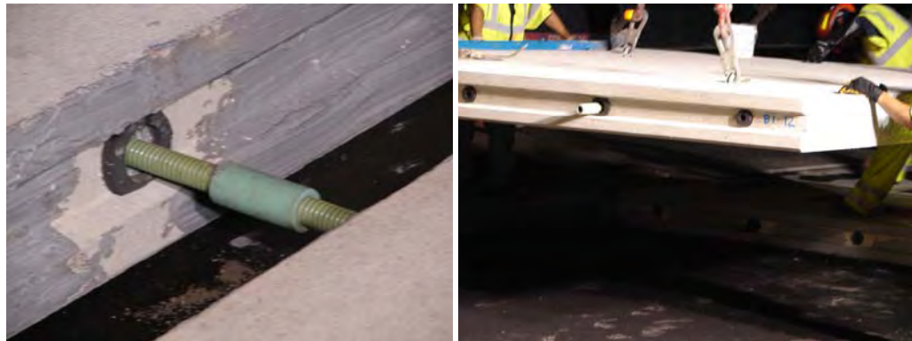
Figure 12.4. Gasket placed on tendon duct.
