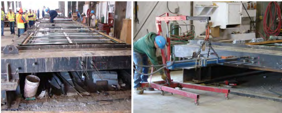
Figure 9.8. Pre-tensioning process.
