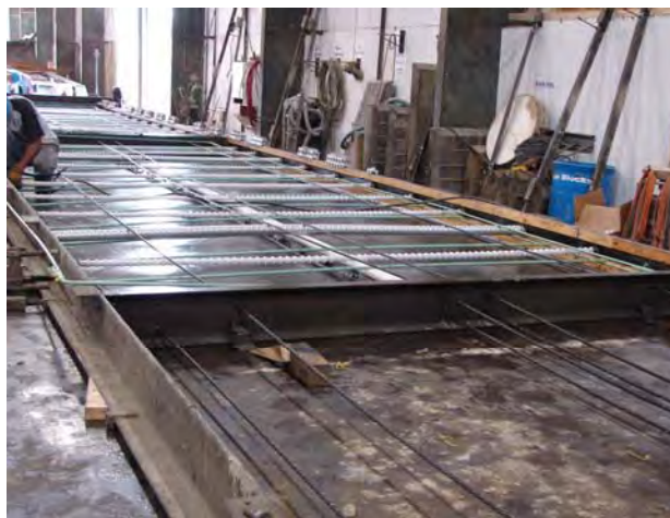
Figure 9.2. Formwork modified to allow for pre-tensioning strands.
