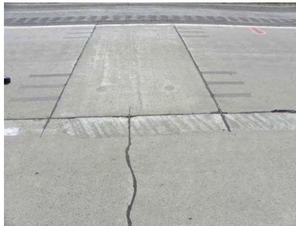
Figure 3.7. View of a well-performing panel at the I-675 project.
