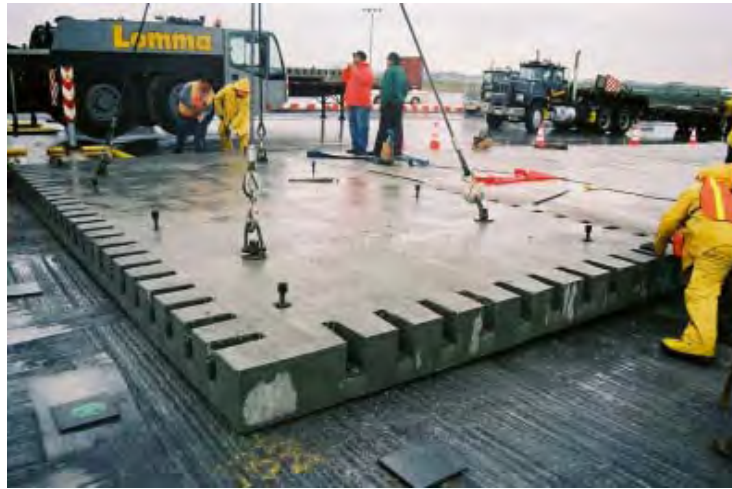
Figure 11.4. Panel placement using setting bolts.
