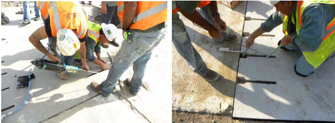
Figure 14.6. Narrow-mouth dowel slot use for repair applications.
