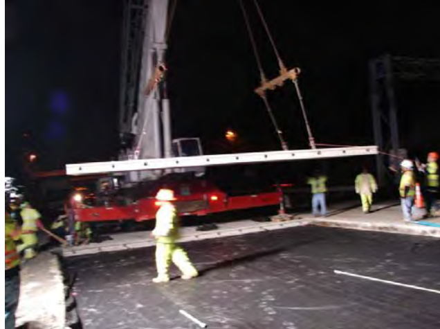
Figure 12.2. Panel placement.
