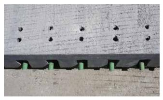
Figure 12: Installation of bottom slot Super Slab® system.
