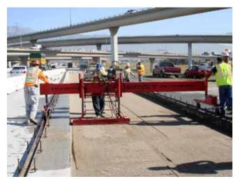
Figure 7: Precision grading for the Super-Slab® System.
