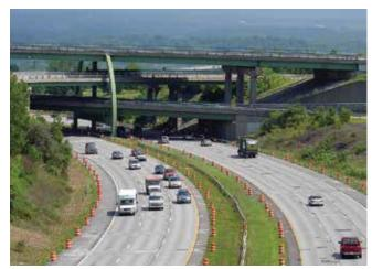
Figure 4: JPrCP installed intermittently in horizontal curves.
