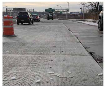
Fiigure 2: Precast slabs installed in frigid conditions – see ice in foreground.
