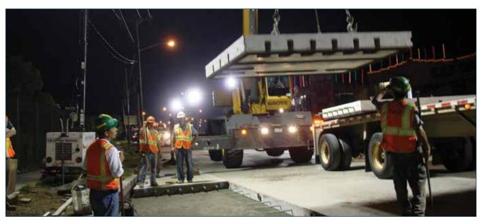
Figure 5: JPrCP installed in a pavement widening during overnight work windows.
