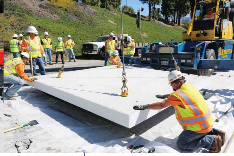
bridges for decades—now its time in roadway reconstruction apparently has come. The I-710 project involves 36 lanemiles of concrete panels, equivalent to 831,000 sq ft or 27,700 cu yd. Among the application's various challenges is the fact that, because of the roadway's geography, the panels taper in width from 26 ft on one end to 36 ft on the other. "Each panel has to get slightly larger so each one is different," Stahl said.
