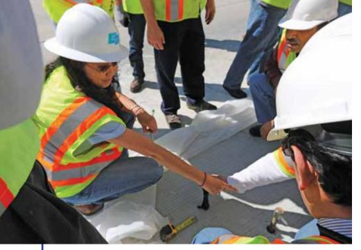
The key to the increased competence is a piece of hardware called (for lack of a better term) a leveling lift, developed by a Caltrans maintenance supervisor. Essentially, it allows the panel to be raised up and down using a screw-like mechanism.
