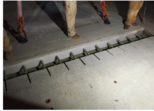
b) Panel installation
