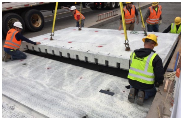
Figure 6. Photo. A PCP panel with dowel bar slots at the bottom.
