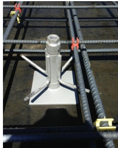
b) Panel leveling lift hardware
