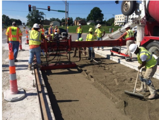
Figure 4. Photo. Cement-treated bedding layer placement.
