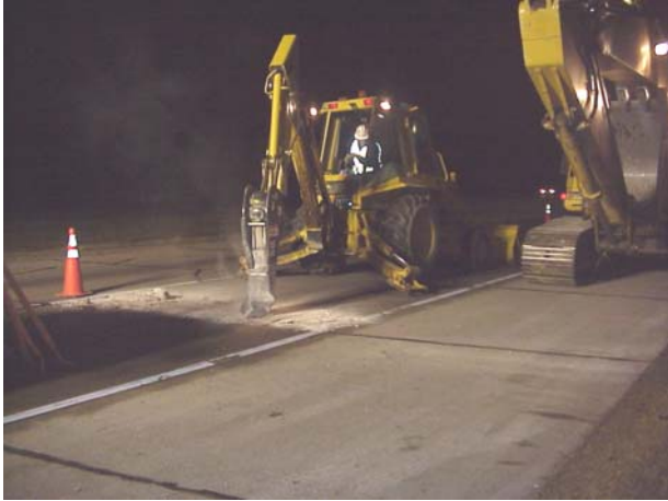
a) Slab demolition
