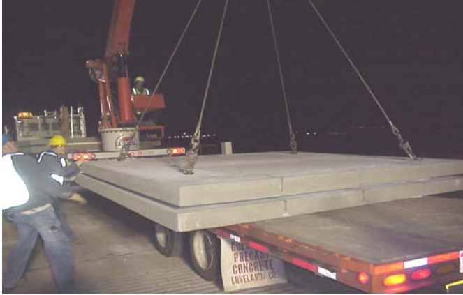
a) Panel moved from flatbed truck.
