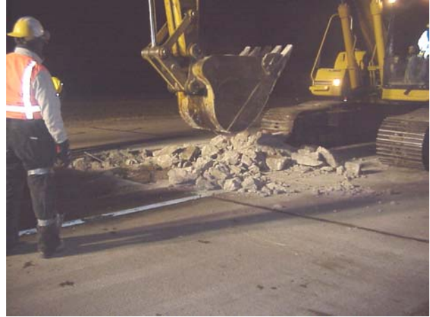
b) Removal of debris
