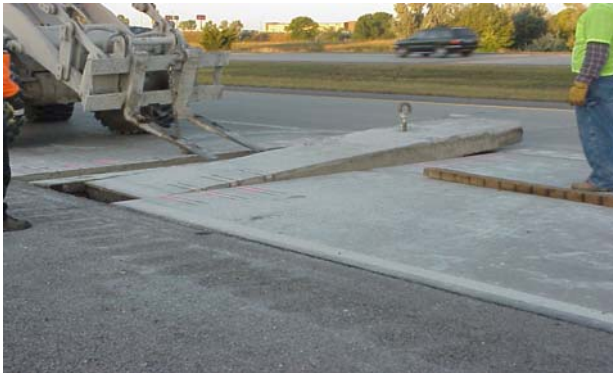
c) Removing the existing slab.
