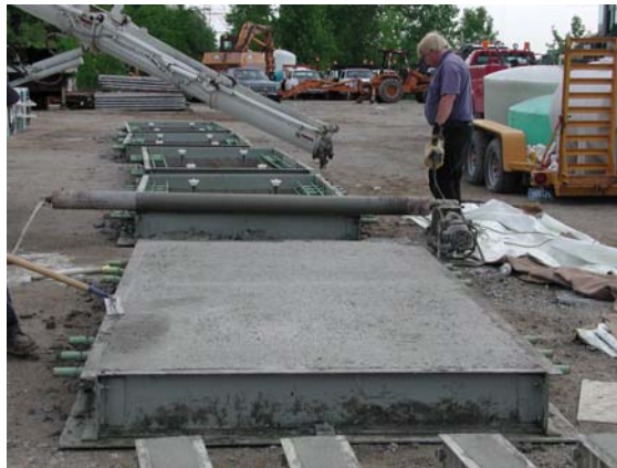
c) Texturing of fresh concrete.
