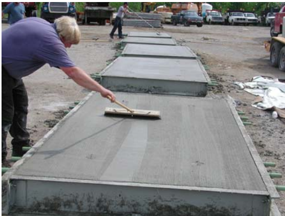
b) Concrete placement for precast panels.
