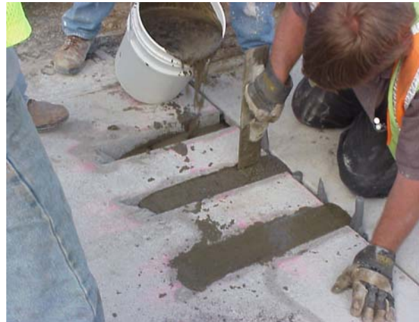
b) Leveling of flowable fill.
