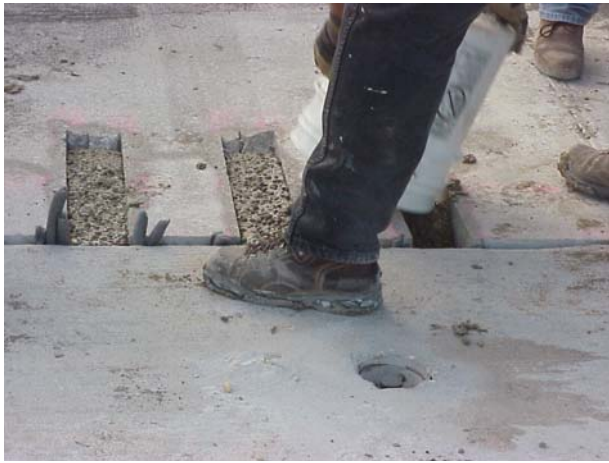
c) Back filling of dowel slots.
