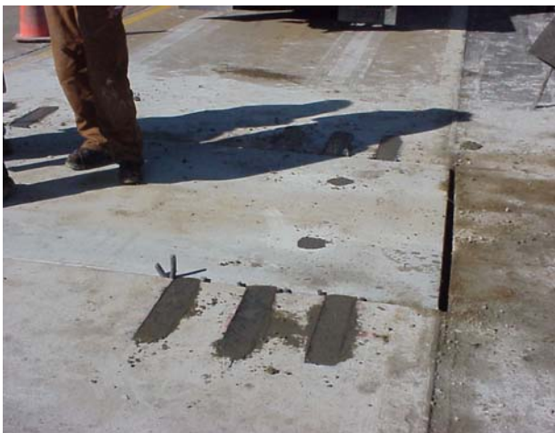
d) Back-filled dowel slots.
