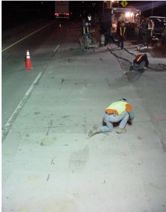
Figure 26. Completed cluster of panels.
