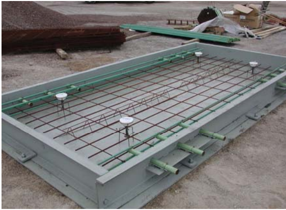
a) Reinforcement and dowel bar placement in the formwork.
