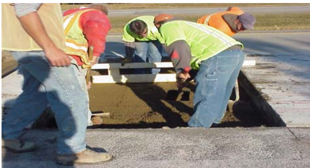
Figure 5. Initial cleaning and preparation of the base.
