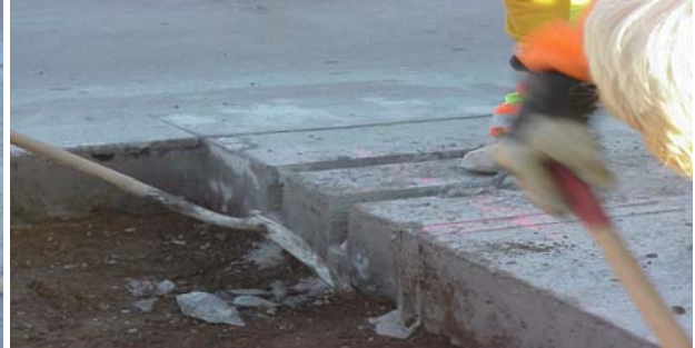
b) Debris removal from dowel slots.
