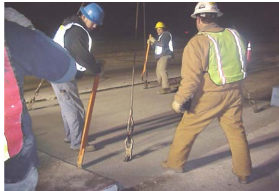
c) Alignment of panel.
