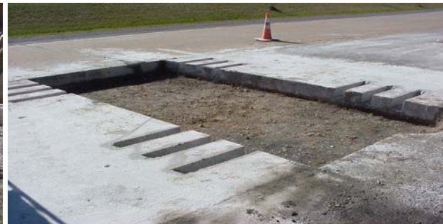
d) Completed dowel slots.
