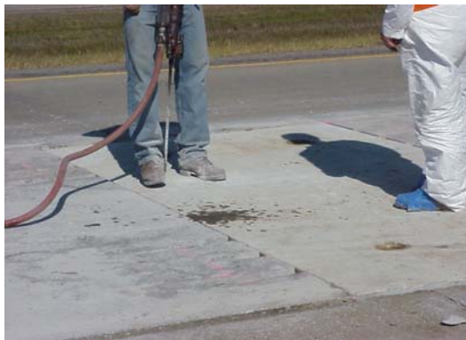
c) Drilling of injection portholes.
