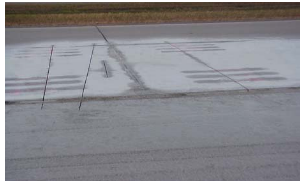
b) The existing slab after sawcutting.
