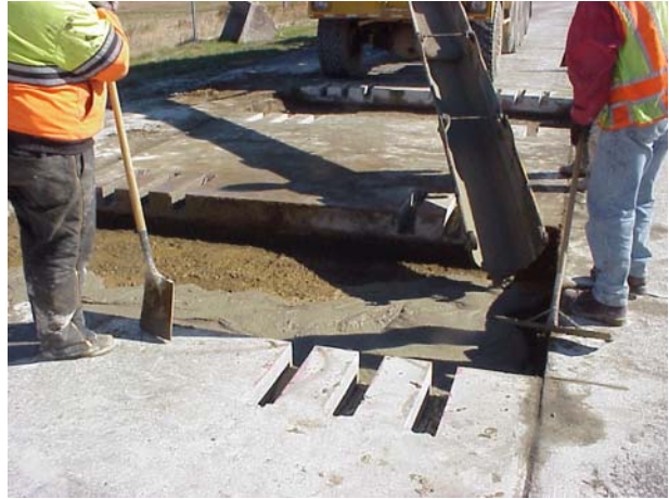
b) Leveling of flowable fill.
