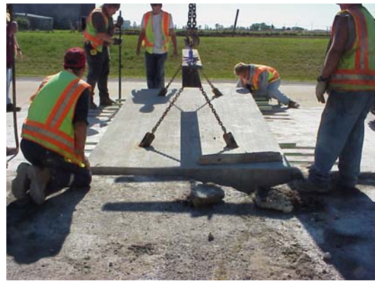
b) Panel installation and alignment.
