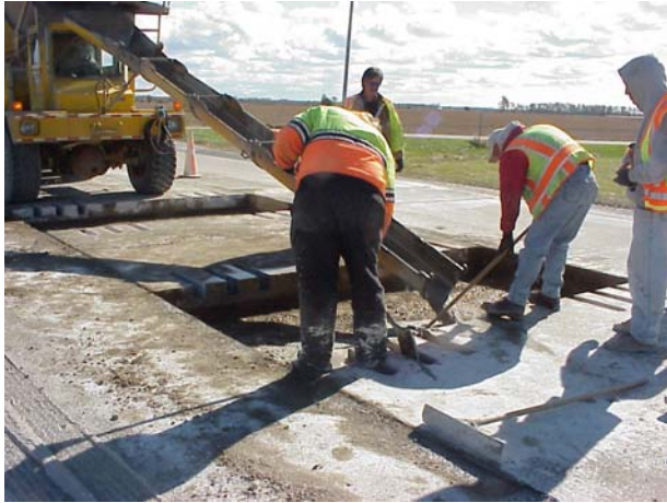
a) Placing of flowable fill.
