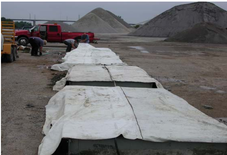
d) Curing of precast slabs.
