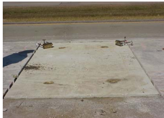
d) Stabilized slab.
