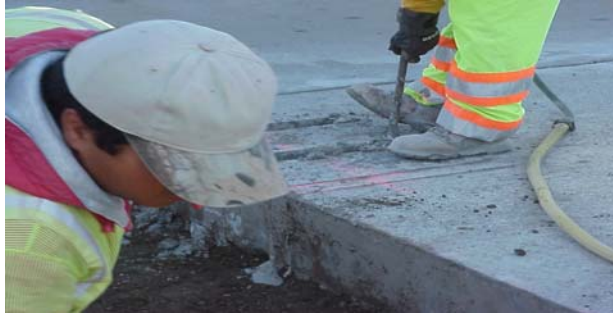
a) Jackhammering of dowel slots.
