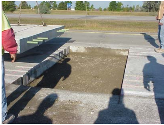
a) Panel installation.
