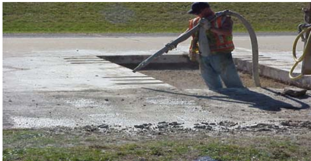
c) Sandblasting of dowel slots.
