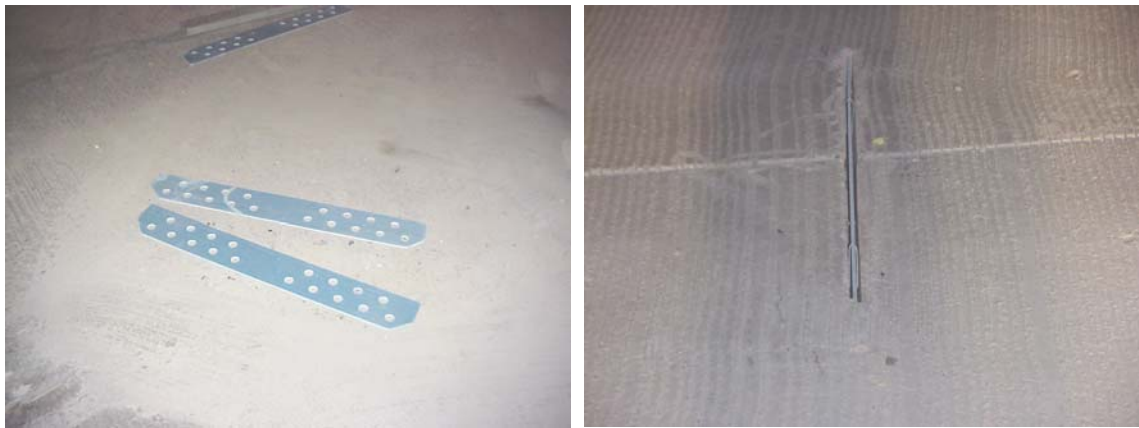
Figure 25. Fiberglass stitches.
