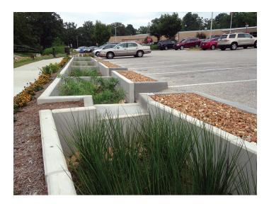
act as temporary storage for runoff water, helping minimize discharge rates. A percentage of water captured also provides irrigation for the vegetation in the planters, further contributing to the overall reduction in the volume of stormwater runoff.
