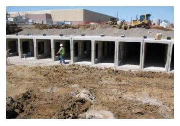
high external loads. After installation, precast retention/detention systems offer maintenance access inside with clear spans and open galleries where workers can remove debris and other sediment that can collect throughout the life of the system.
