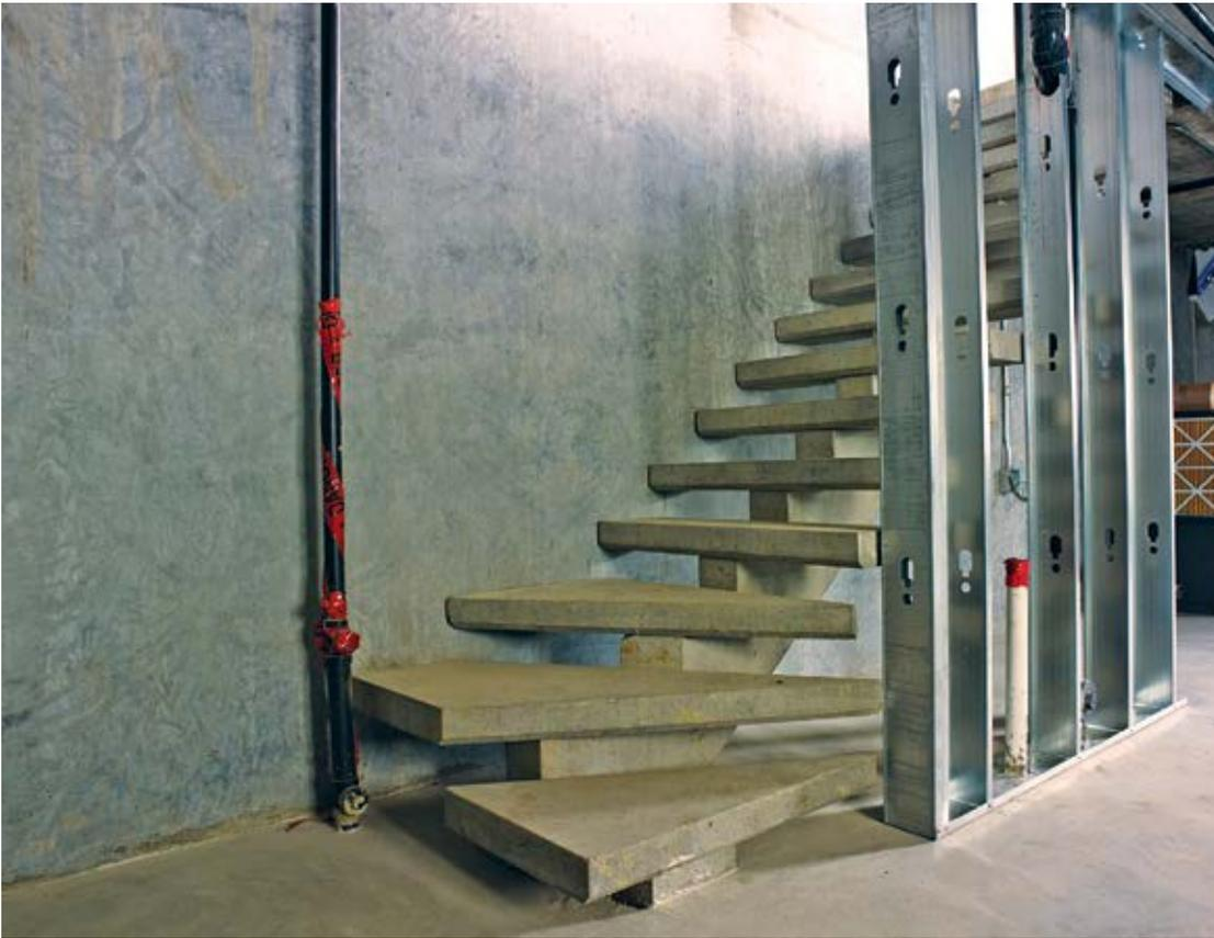
◀ Precast concrete is featured on the interior as well in the form of cantilevered precast stair treads. Photos courtesy of Ian Grant Photography
