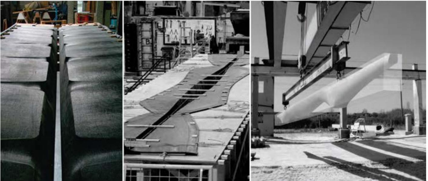
*(left) Fabric formwork for a 16.5-ft variable section T-beam constructed by Ronnie Araya, architect.*
