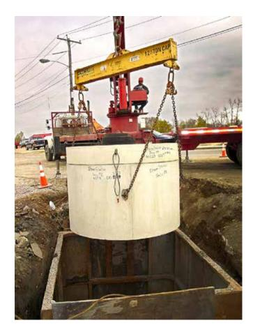
be designed to prevent all infiltration/exfiltration of the manhole. Consult ASTM C443 for watertight joints. Storm manholes on the other hand should be designed to prevent soils from filtering into the system, but do not typically require complete watertight joints. Consult ASTM C990 for soil-tight joints.
