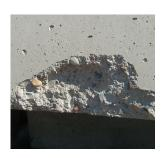
reinforcement (also known as pinning) and using a build-up application technique. This will be discussed under the section on spalls. Most chips can be repaired in one application with the appropriate patching material.
