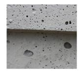
especially with architectural finishes. The common causes of bugholes include entrapped air, water pockets or the improper application of form release agent.
