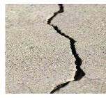
the crack is acceptable, needs remediation or cannot be repaired. Cracks should be sealed when necessary to prohibit premature deterioration or shorten service life of the product.
