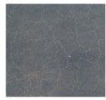
the curing process. Crazing can be avoided by using curing compounds, covering the product during curing, refraining from "over-finishing" the surface of the concrete, and not finishing the product while bleed water is still present on the surface. Crazing cracks are typically not repaired because they are not structural and they are so small that it would be nearly impossible to fill them with any material.
