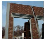
reinforcement around the blockout will be reduced, therefore, additional design considerations need to be addressed. Sometimes this situation may require additional external connections to relieve stress on the piece, strong backs or modification to the piece.
