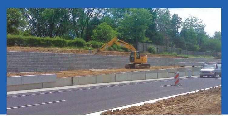
sides of the roundabout – the initial bid was for only one of the four walls – using block ranging from 24 in. deep to 60 in. deep. The product met all time, budget and location constraints, minimized excavation and required no soil reinforcement. "All parties were so relieved," Fouts said. "It's just such a great solution."
