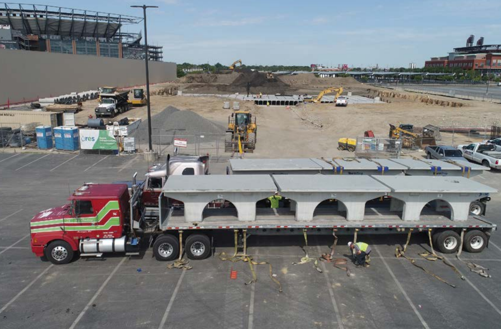
A precast concrete stormwater detention system helps manage runoff near the home of the Philadelphia Eagles and Phillies. Designers chose precast concrete for its durability and an easy installation.
