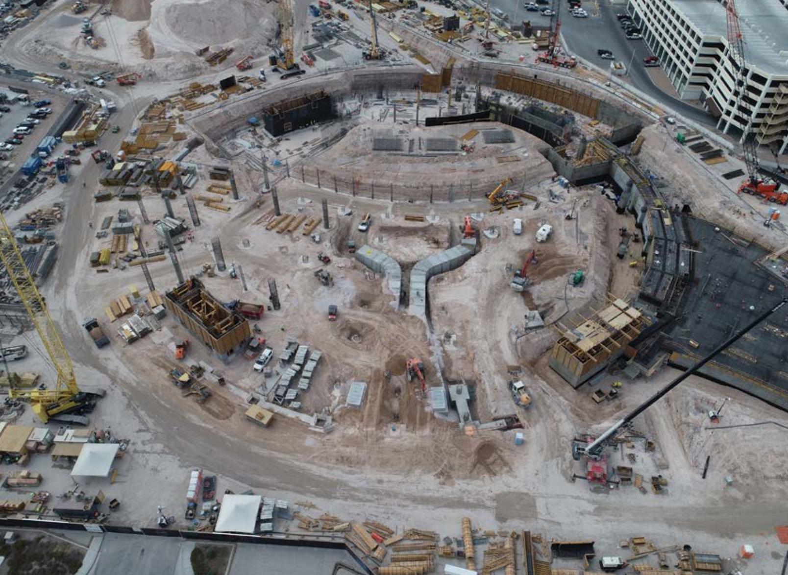
More than 100 precast concrete box culvert sections provide the air duct system for a new building in Las Vegas.
