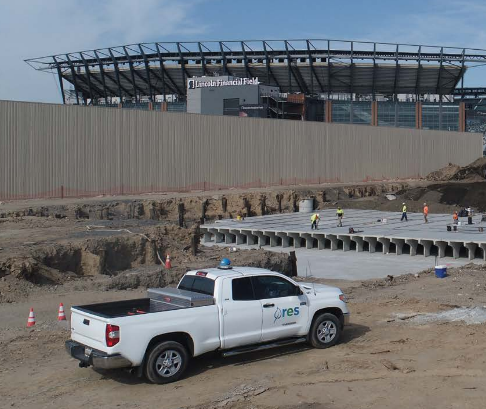
Challenging soil conditions and load-bearing capacity led designers to choose precast concrete.
