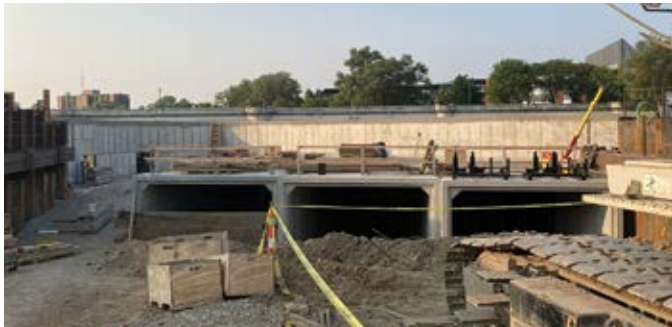
Due to the job site's location beneath a city park, officials turned to precast concrete.
