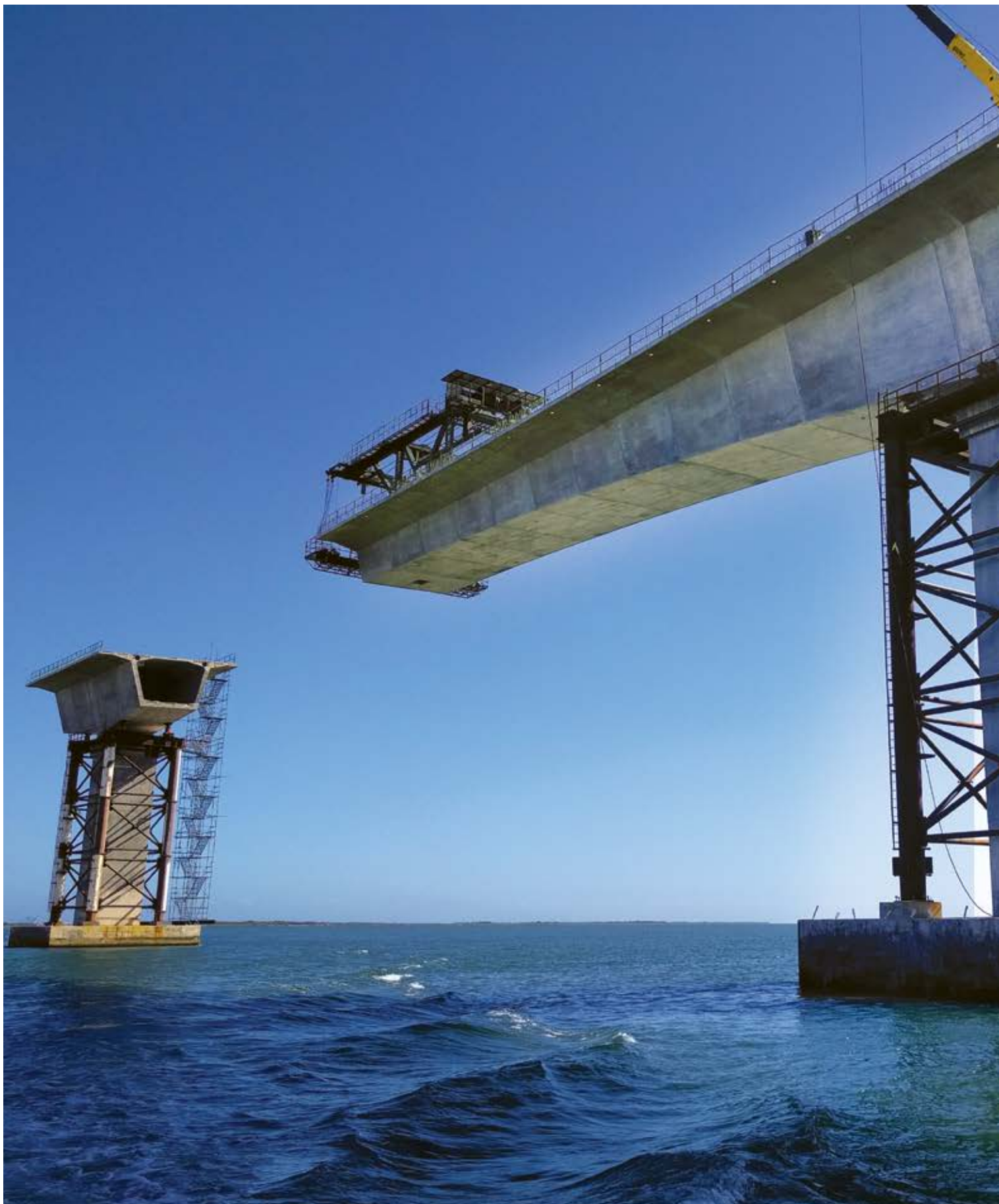
The massive structure includes nine 350-foot spans.
