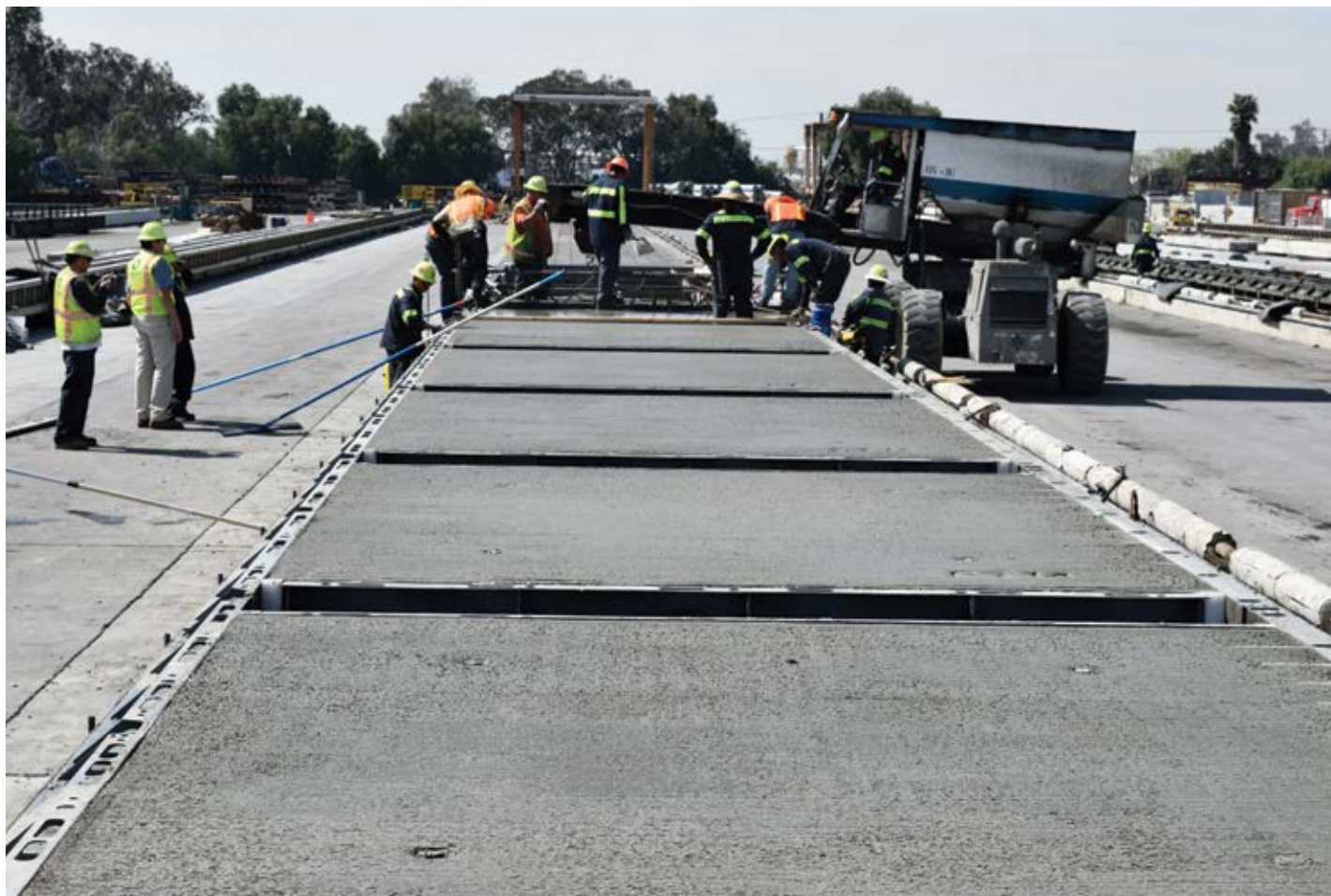
Panels were fabricated in a new, 500-foot self-stressing bed.
