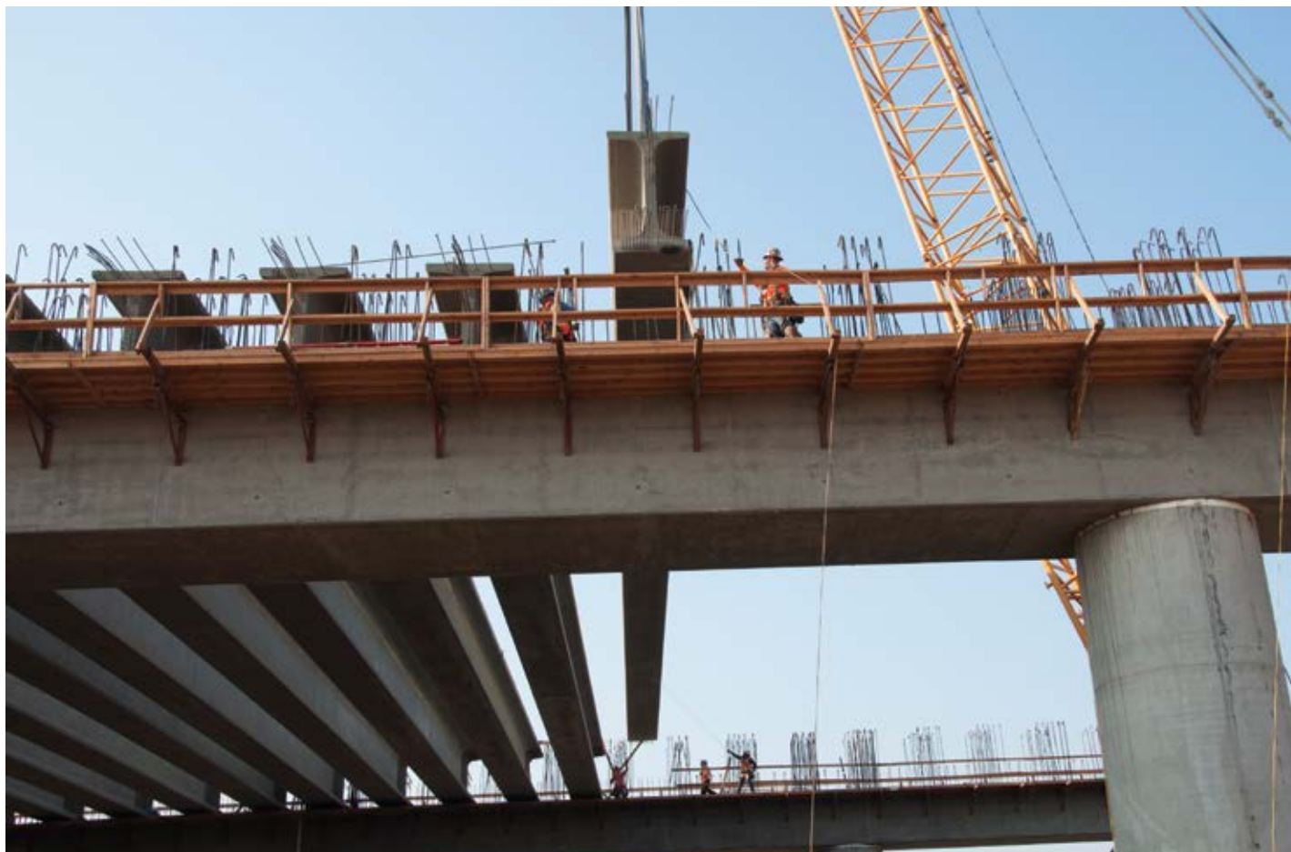
Project precaster Con-Fab California is manufacturing more than 2,000 precast concrete components for the HSR project.
