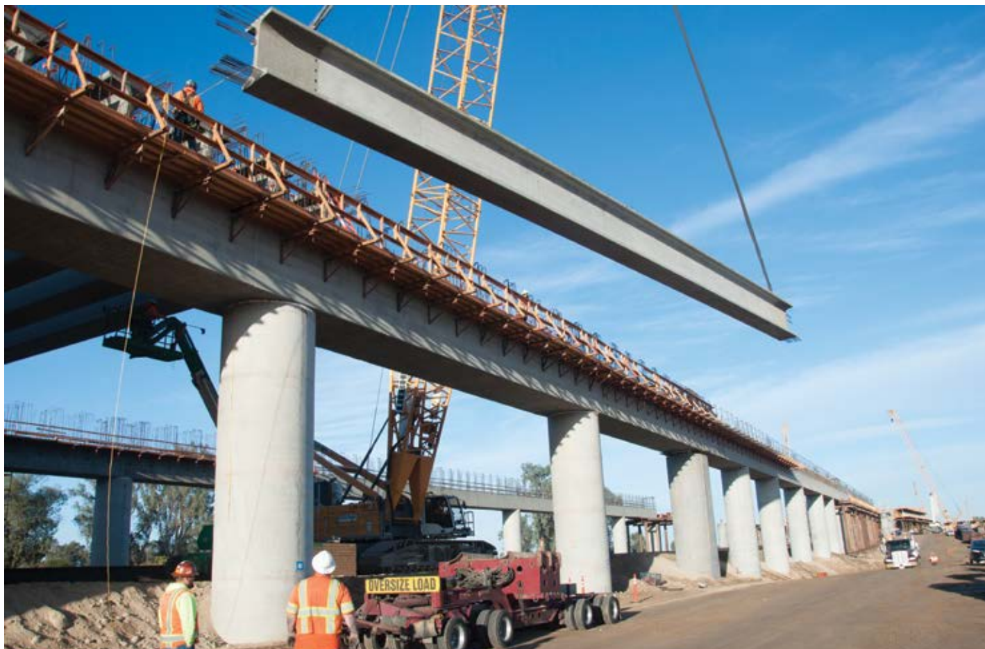
Joint venture firm Tutor Perini/Zachry/Parsons selected precast concrete to save time and increase efficiency on the California High-Speed Rail project.
