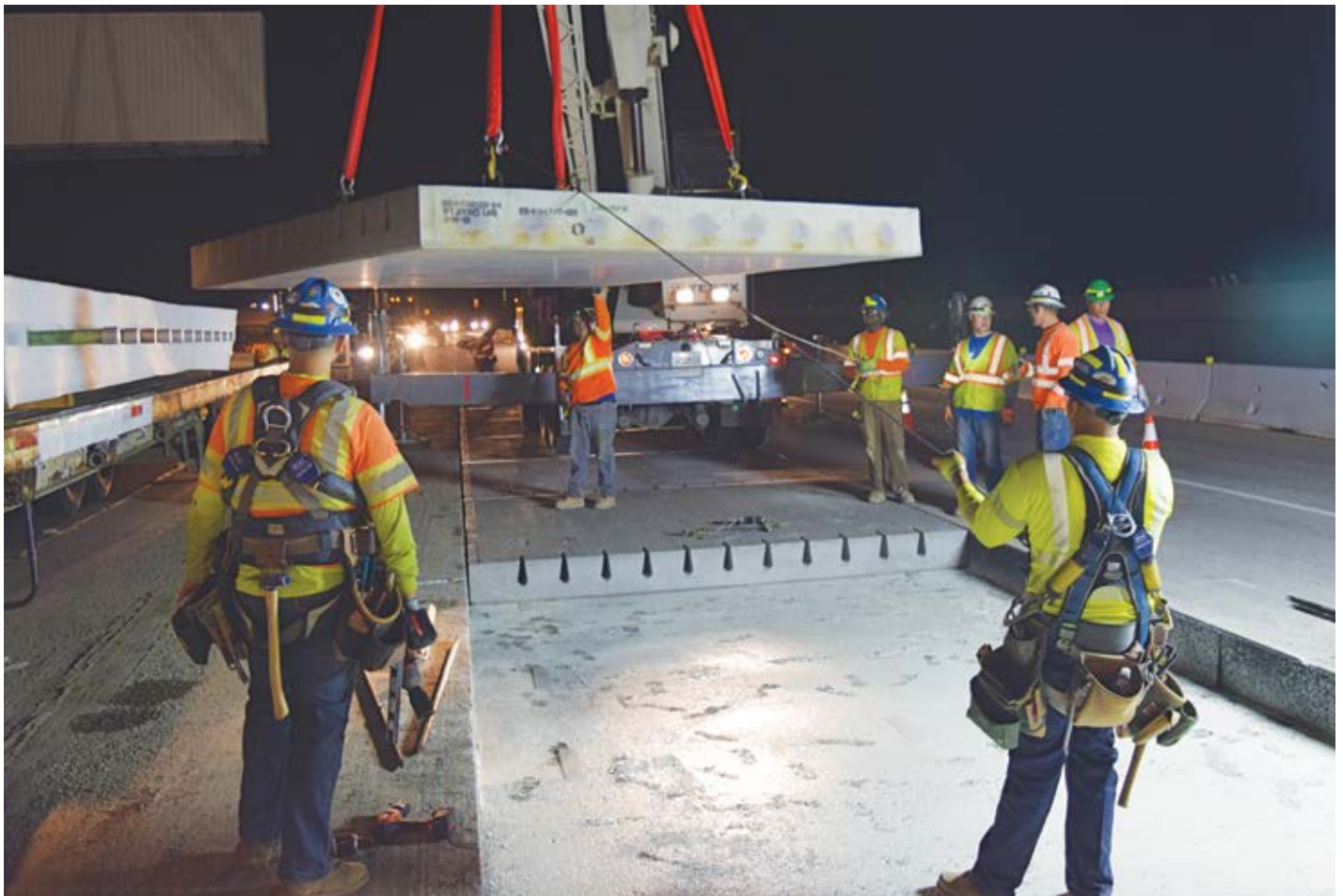
Workers installed the panels during overnight work windows, limiting the impact on traffic.
