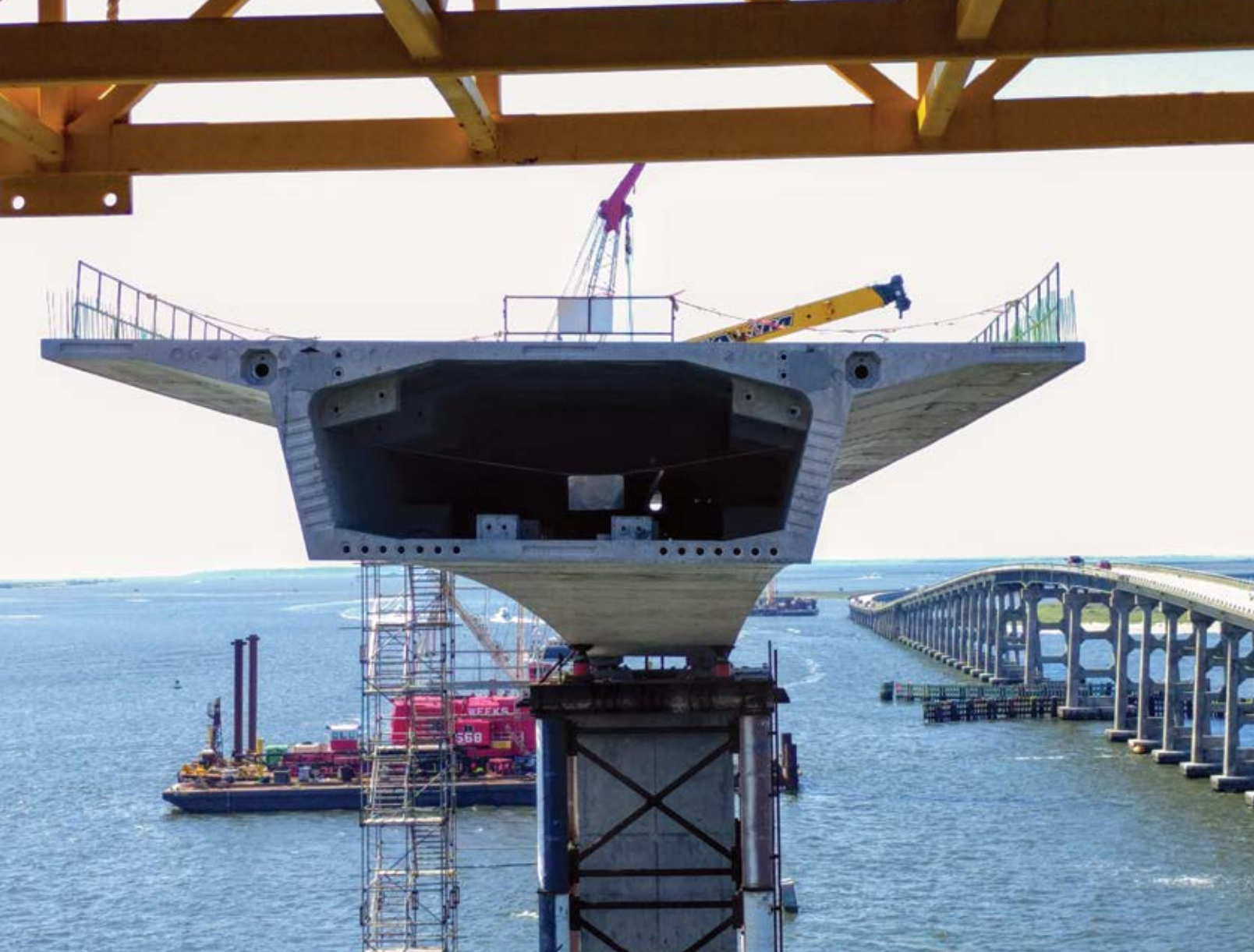
The new Bonner Bridge incorporates a balanced cantilever design featuring a wide variety of precast concrete products.
