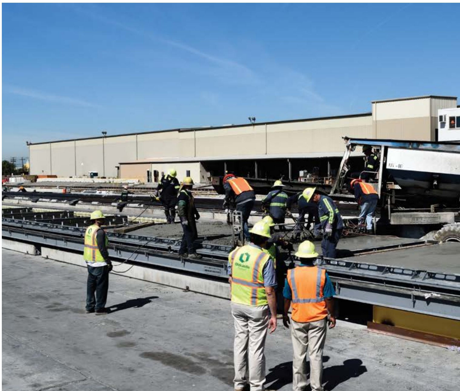
Oldcastle Precast manufactured 6,500 precast concrete pavement panels for the Foothill Freeway project in California.
