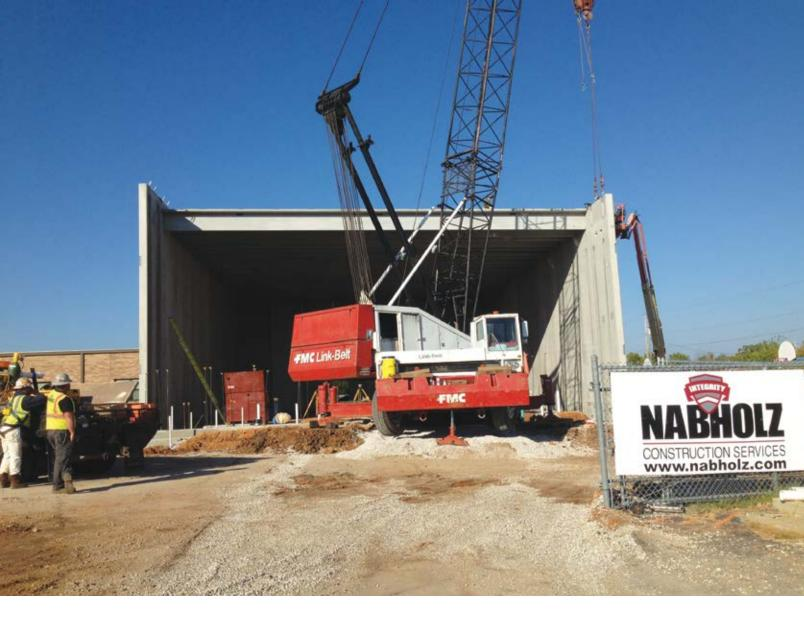
Nabholz Construction Services. The remaining two shelters are in the final stages of design. A prestressed concrete construction with numerous special connections and reinforcing make up the shell.
