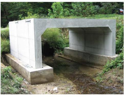
for road width) above narrow streams. The height of the box culvert is dependent on amount of flow and site conditions.
