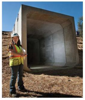
It is popular where there are environmental issues or a desire to avoid disturbance to a stream bed. This structure can sit on a CIP footing situated on opposite sides of a stream. The three-sided arch spans the stream without adversely affecting the stream's natural state.
