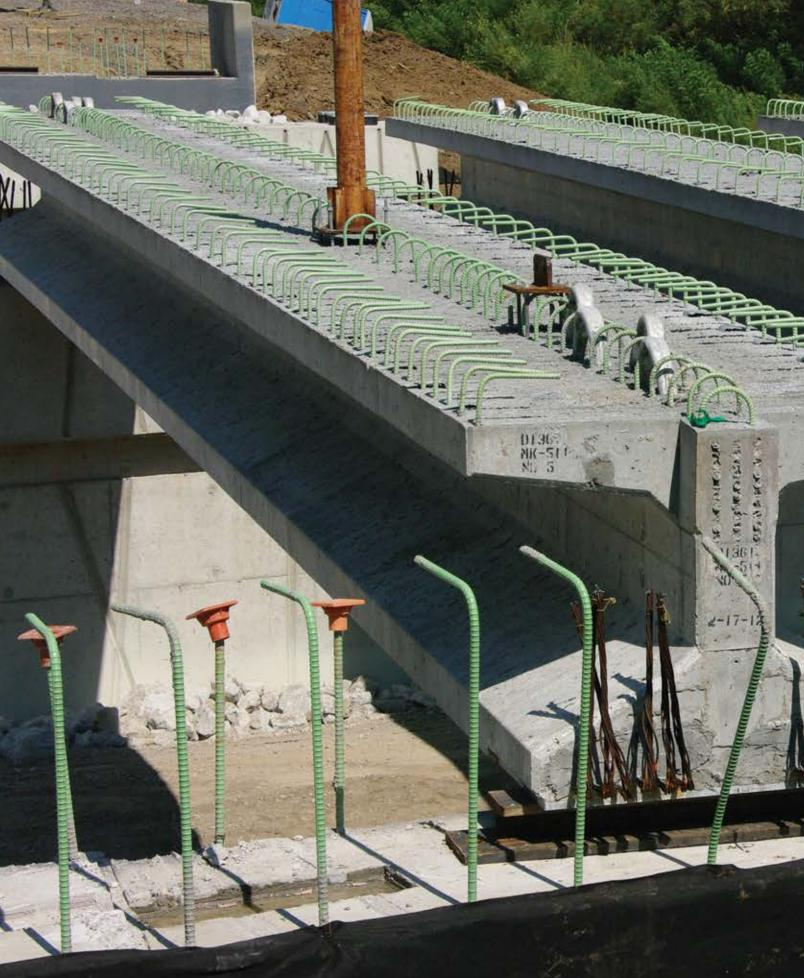
The hybrid Bulb-T bridge beam has a shallower shape for a more efficient use of material.
