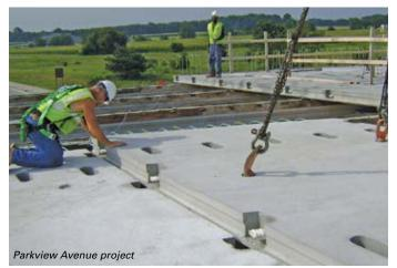
the beams to ensure a smooth transition at the closure pour joint. High Performance Superstructure Concrete (HPSC), capable of attaining 7,000 psi compressive strength, was used for the closure pours between beam-deck segments. Transverse post-tensioning tendons comprised of four ½-in.-diameter strands were installed in 5-in. ducts cast into the six diaphragms of the modular sections, stressed to 182 kips and grouted with HPSC.
