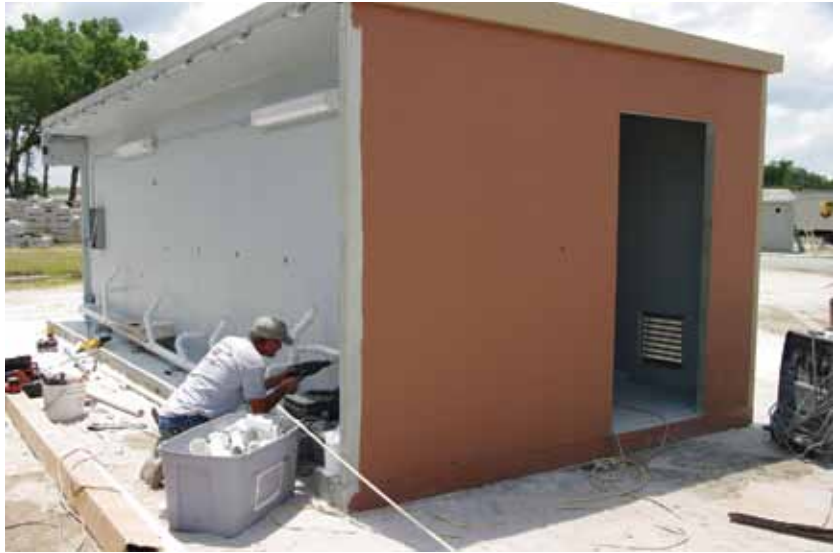
Plumbing and electrical fixtures can be added at the plant, saving installation time on site.
