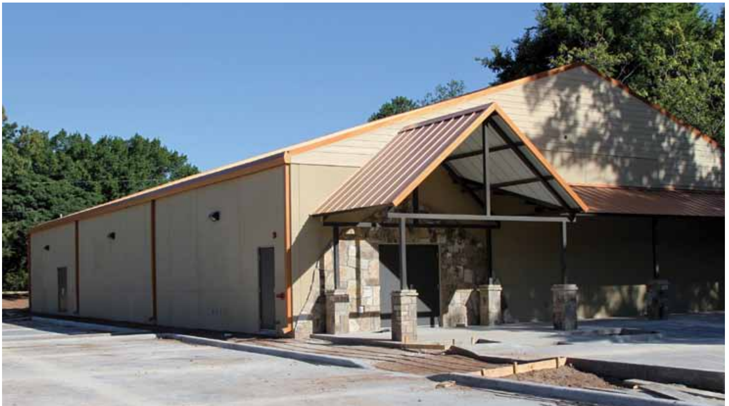
Precast concrete community center in Emory, Texas, designed by Speed Fab-Crete to withstand winds in excess of 250 mph (an F5 tornado).
