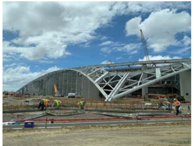
Photo courtesy of Euclid Chemical Co.
