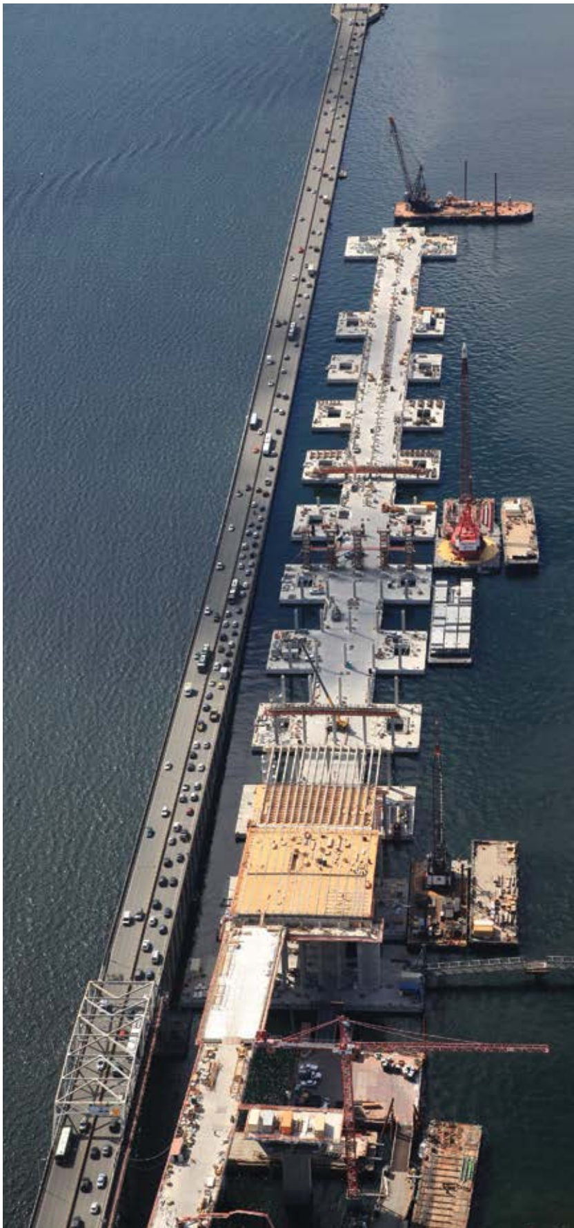
The SR520 Floating Bridge between Seattle and other communities on Lake Washington was the world's longest floating bridge when it opened in 2016, replacing a 1963 structure, and was built to withstand a 100-year storm.
