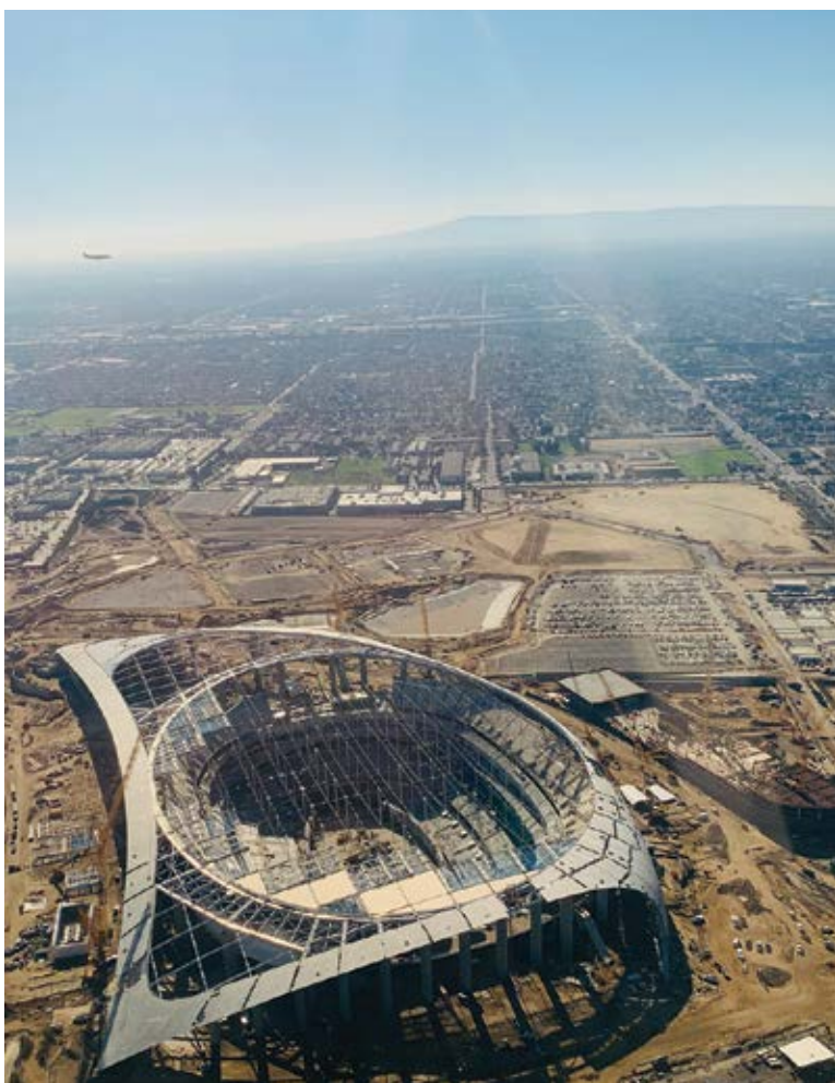
Photo courtesy of Euclid Chemical Co.
