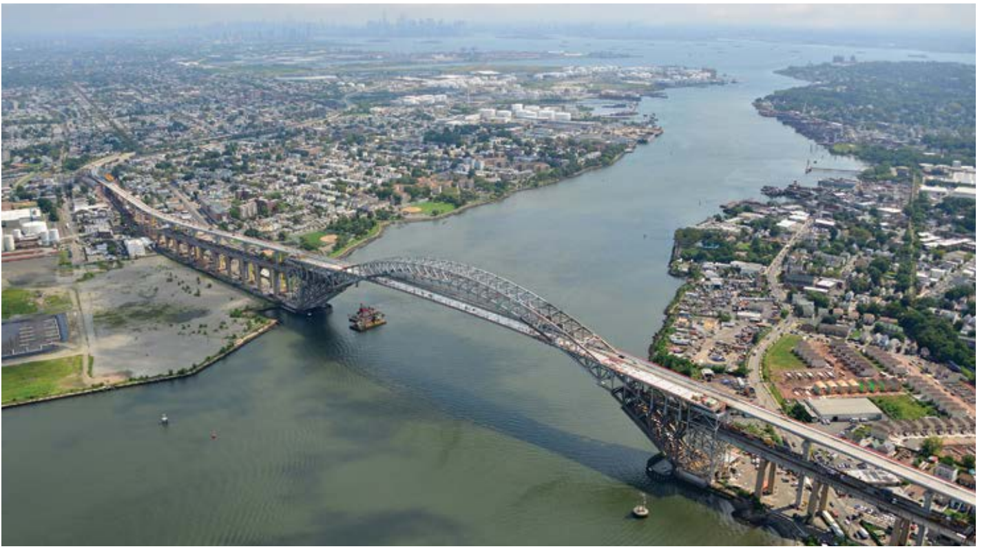
The substructure and superstructure of the Bayonne Bridge are both precast, post-tensioned concrete, making it a one-of-a-kind structure.
