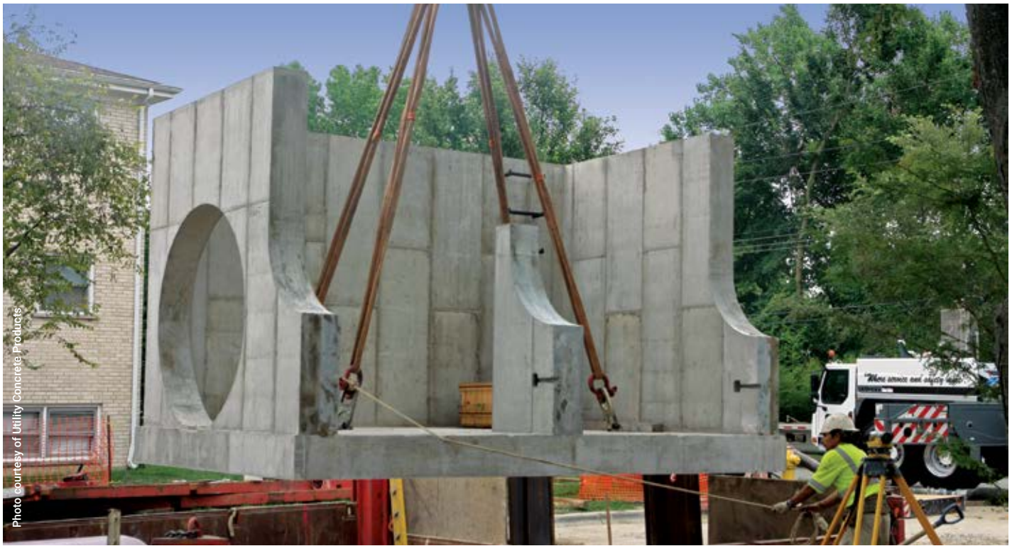
Six custom precast concrete units create a massive utility junction in Illinois. Installation of the junction took only 2.5 hours, minimizing disruptions to area residents.
