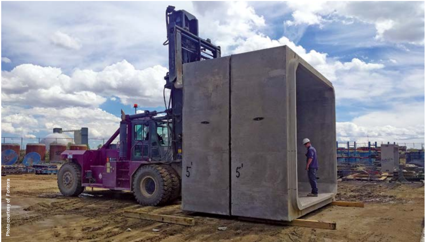
Precast concrete is at the heart of Denver's largest-ever stormwater drainage project.
