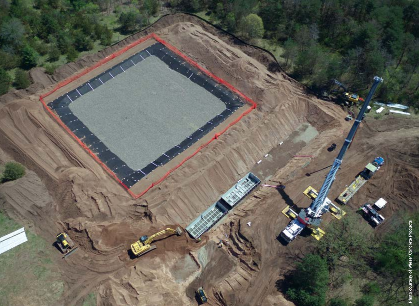
Minnesota's largest on-site decentralized wastewater treatment plant features five 38,000-gallon and four 10,000-gallon precast concrete tanks.
