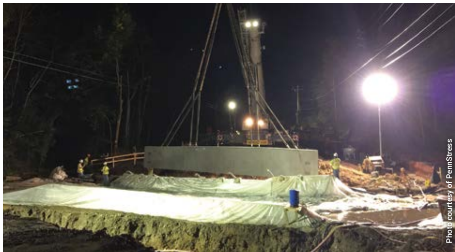
Crews were able to replace the bridge in a mere eight days thanks to the use of precast concrete materials.
