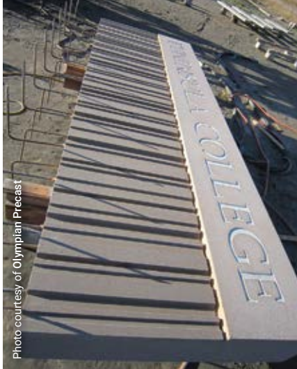
(Above) Olympian Precast produced ribbed precast concrete signs for a local community's multiphase gateway project. (Left) The company also manufactured a monument sign for Peninsula College that included an integral pigment and two different finishes.
