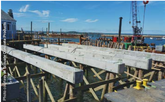
For a wharf replacement project in Plymouth, Mass., Scituate Concrete Products manufactured six massive, 55,000-pound precast beams along with numerous smaller precast slabs and pieces.
