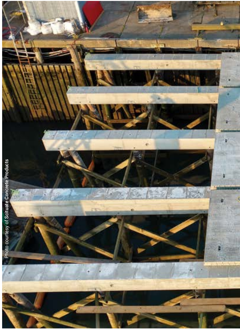
For a wharf replacement project in Plymouth, Mass., Scituate Concrete Products manufactured six massive, 55,000-pound precast beams along with numerous smaller precast slabs and pieces.
