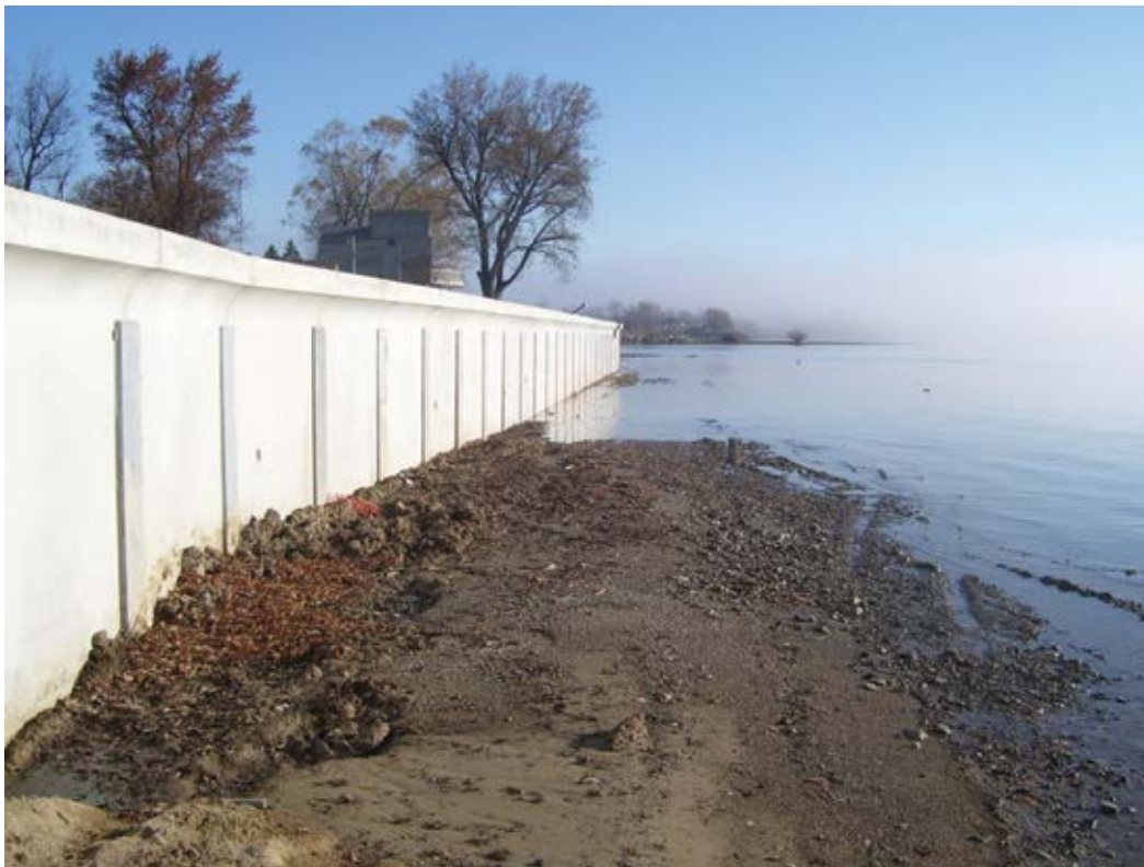
The new precast concrete seawall at Detroit Beach will replace the deteriorating structure currently in place.
