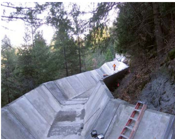
Flume 41 near Riverton, California, now has a 100-year lifespan thanks to lightweight precast.
