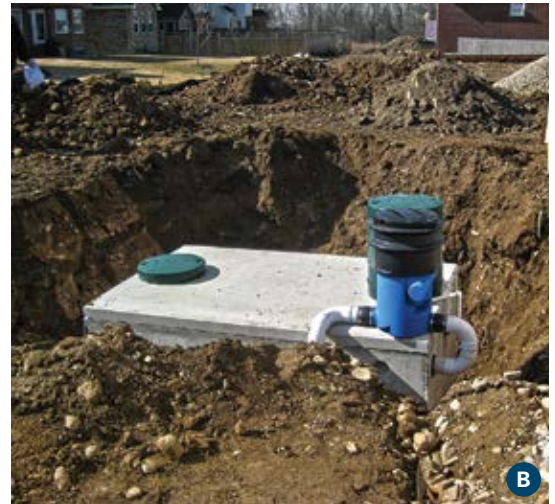
RH20's underground precast rainwater harvesting systems helped reduce overall water discharge flows by 60% for a neighborhood in Newmarket, Ontario.
