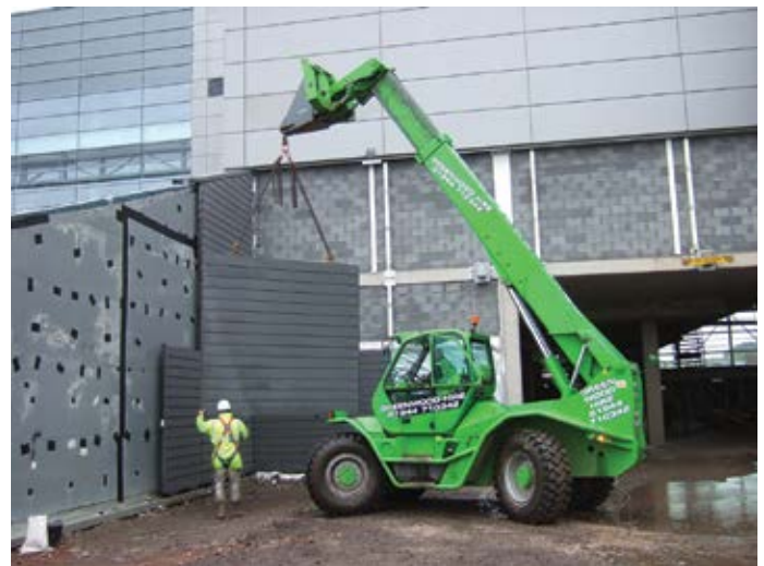
Precast panels are installed on the Emirates Arena in Glasgow, Scotland. Photo courtesy of Decomo UK.JPG
