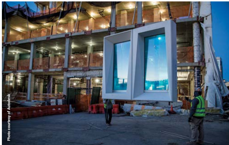
Crews work to install precast concrete panels for One South First in Brooklyn. The panels were designed to mimic sugar crystals as a tribute to the former Domino Sugar Refinery.
