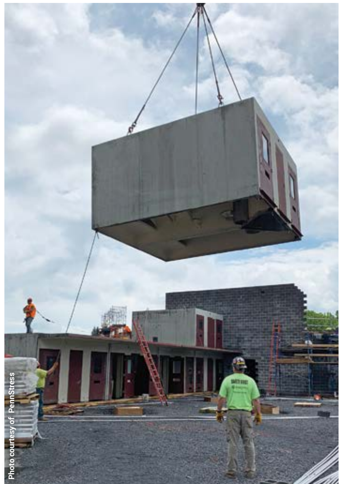
PennStress manufactured 128 precast concrete jail cells. By using precast concrete and modular construction, crews were able to quickly build the correctional facility.
