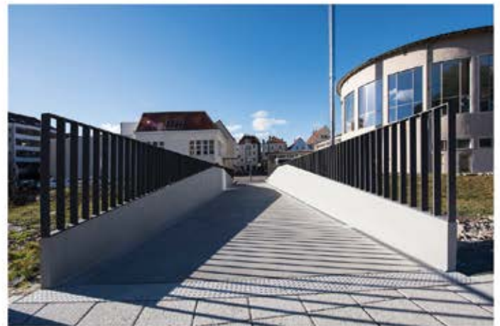
First pedestrian bridge worldwide that is reinforced with only carbon-reinforcements and which contains no steel reinforcement or prestressing steel; Albstadt, Germany, [Max Bögl Group, www.max-boegl.de ], finished in 2015.
