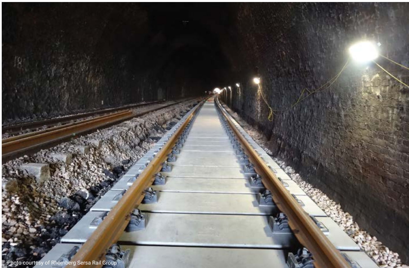
Workers installed approximately 800 feet of IVEs precast slab track at Asfordby Tunnel in the U.K.
