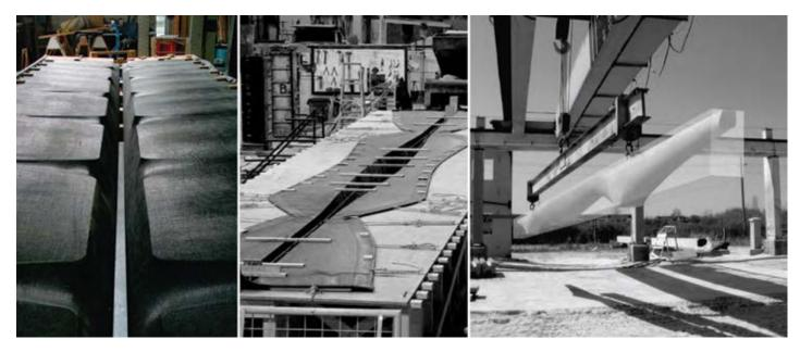
(left) Fabric formwork for a 16.5-ft variable section T-beam constructed by Ronnie Araya, architect.
