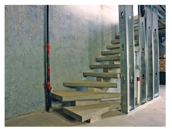
Precast concrete is featured on the interior as well in the form of cantilevered precast stair treads. Photos courtesy of lan Grant Photography
