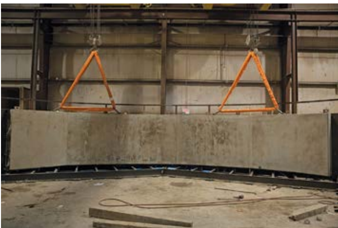
Faddis Concrete Products produced 24 arch leaves to create a bridge that has a horizontal span of 42 feet.
