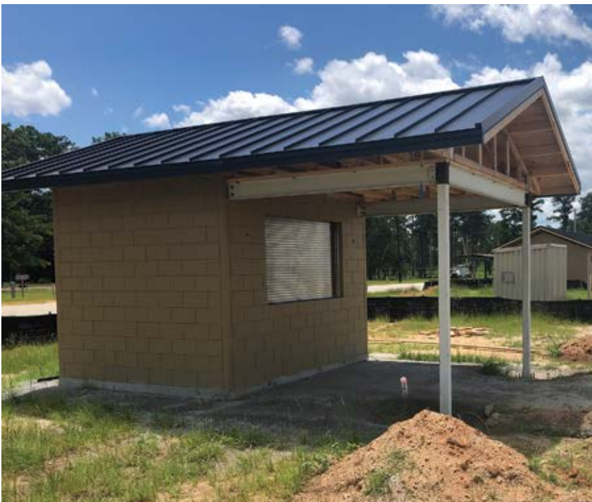
The precast facades were made to look like hand-laid masonry to match the existing architecture. By using precast, the project was completed in just a few months.
