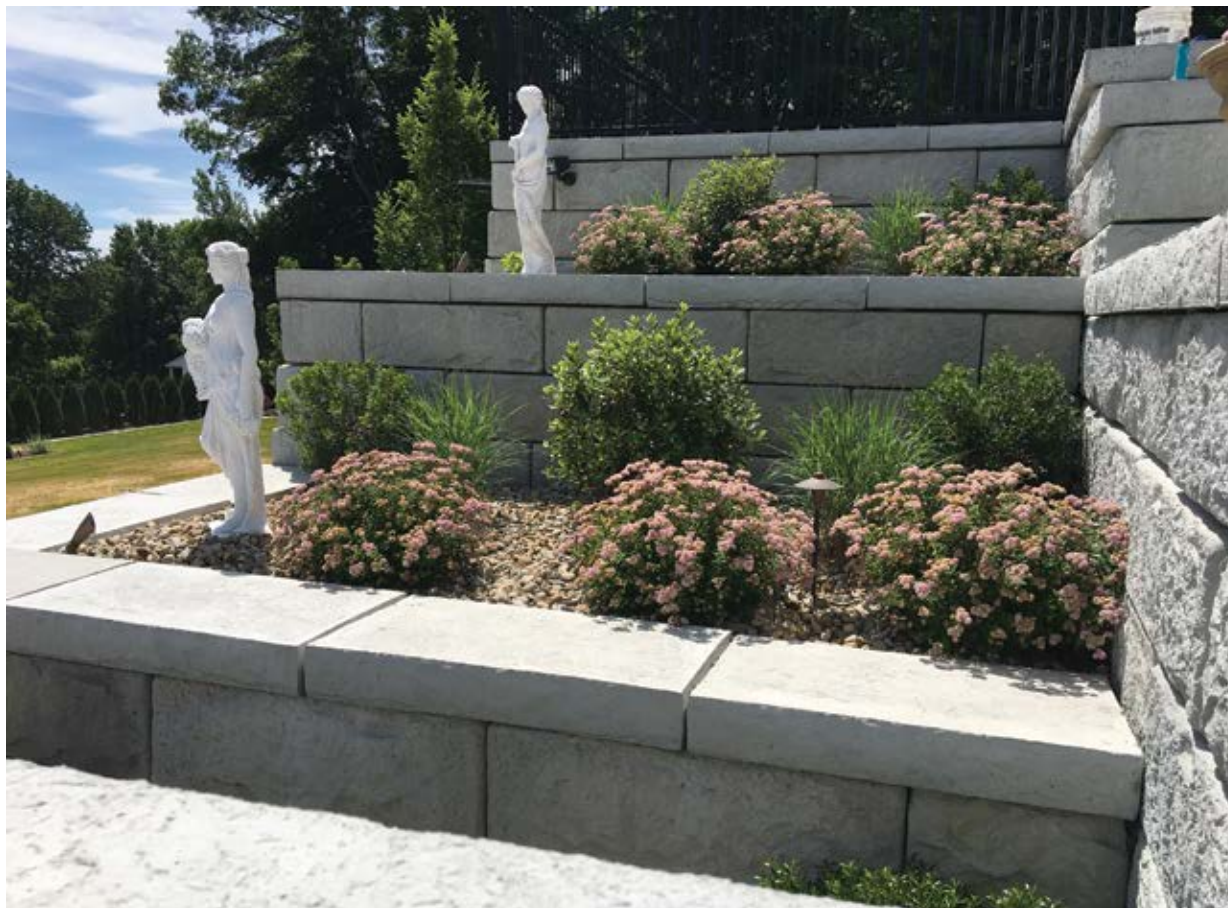
The ReCon blocks were given a granite textured finish to match the aesthetics of the house.
