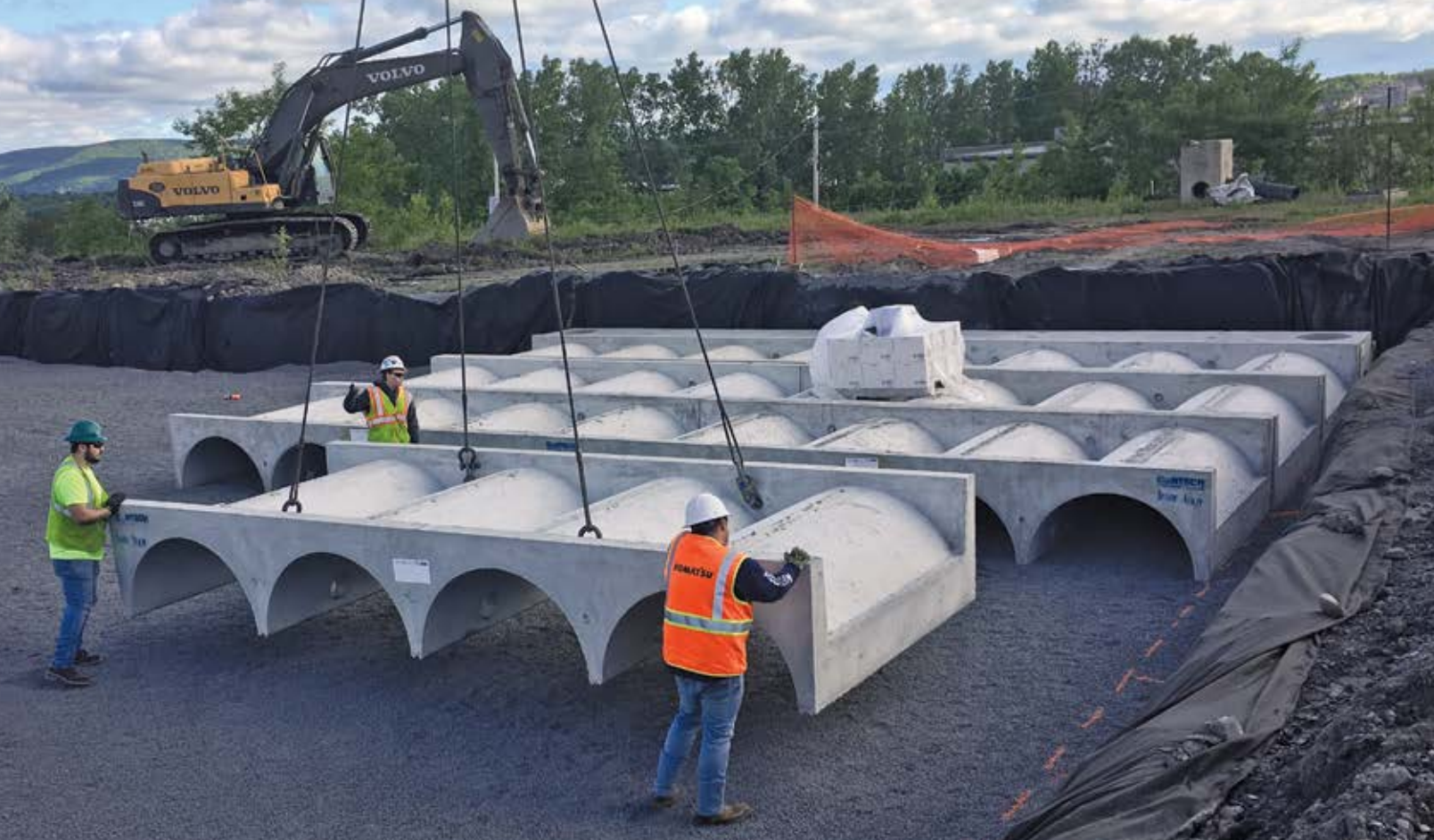
Workers install the Terre Arch 26 stormwater system for an office park in Scranton, Pa. The system was chosen for its quick installation time with the basins being installed in just two days.
