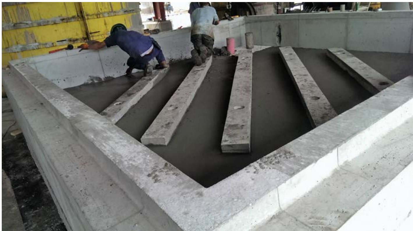
The floor of the custom precast wastewater structure was hand-sloped around 8-inch-by-8-inch support beams at a fixed angle leading to a sump blockout in the floor.
