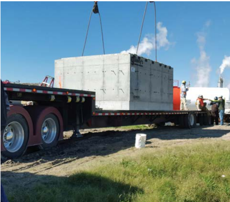
Project contractor Beard Construction completed installation of the precast concrete containment structure in just one day.
