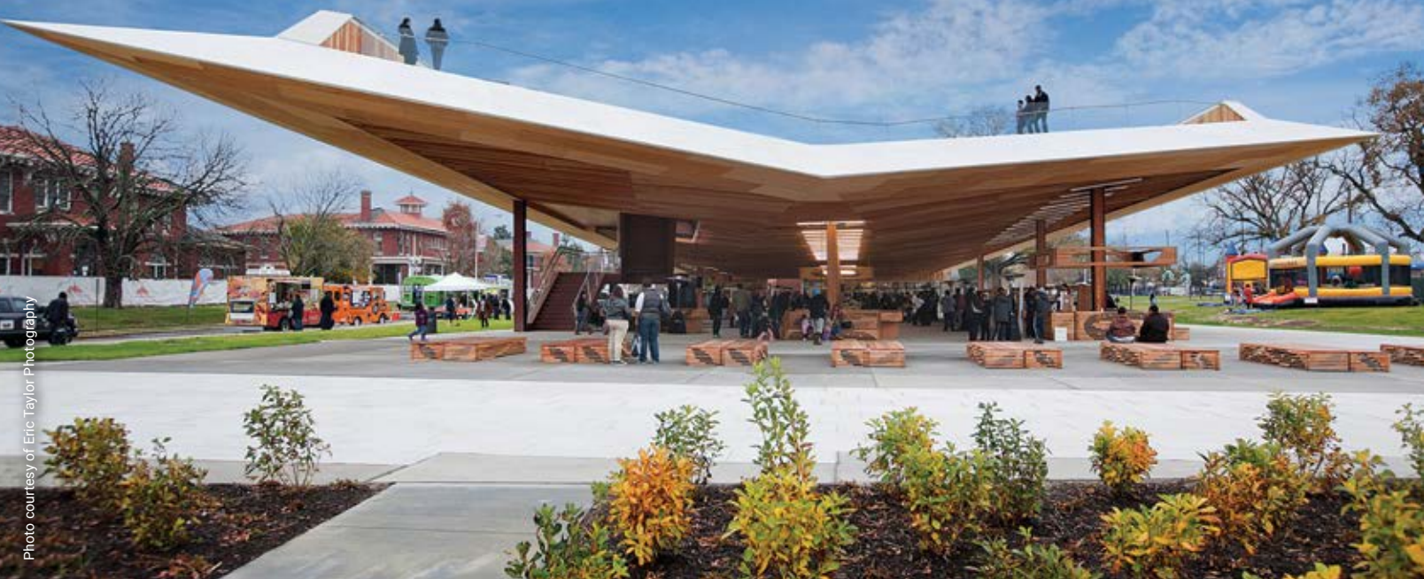
The St. Elizabeths East Gateway Pavilion in Washington, D.C., was constructed with a striking UHPC roof.
