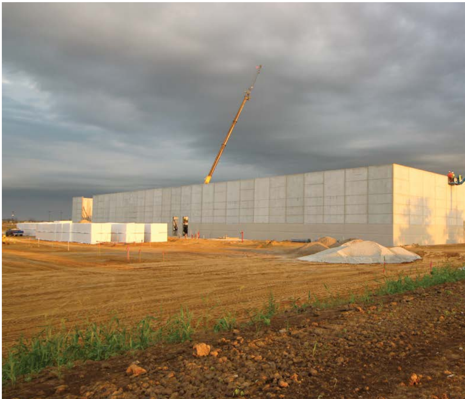
Workers pieced together nearly 100 load-bearing precast concrete panels to construct Jonathan Byrd's Fieldhouse.
