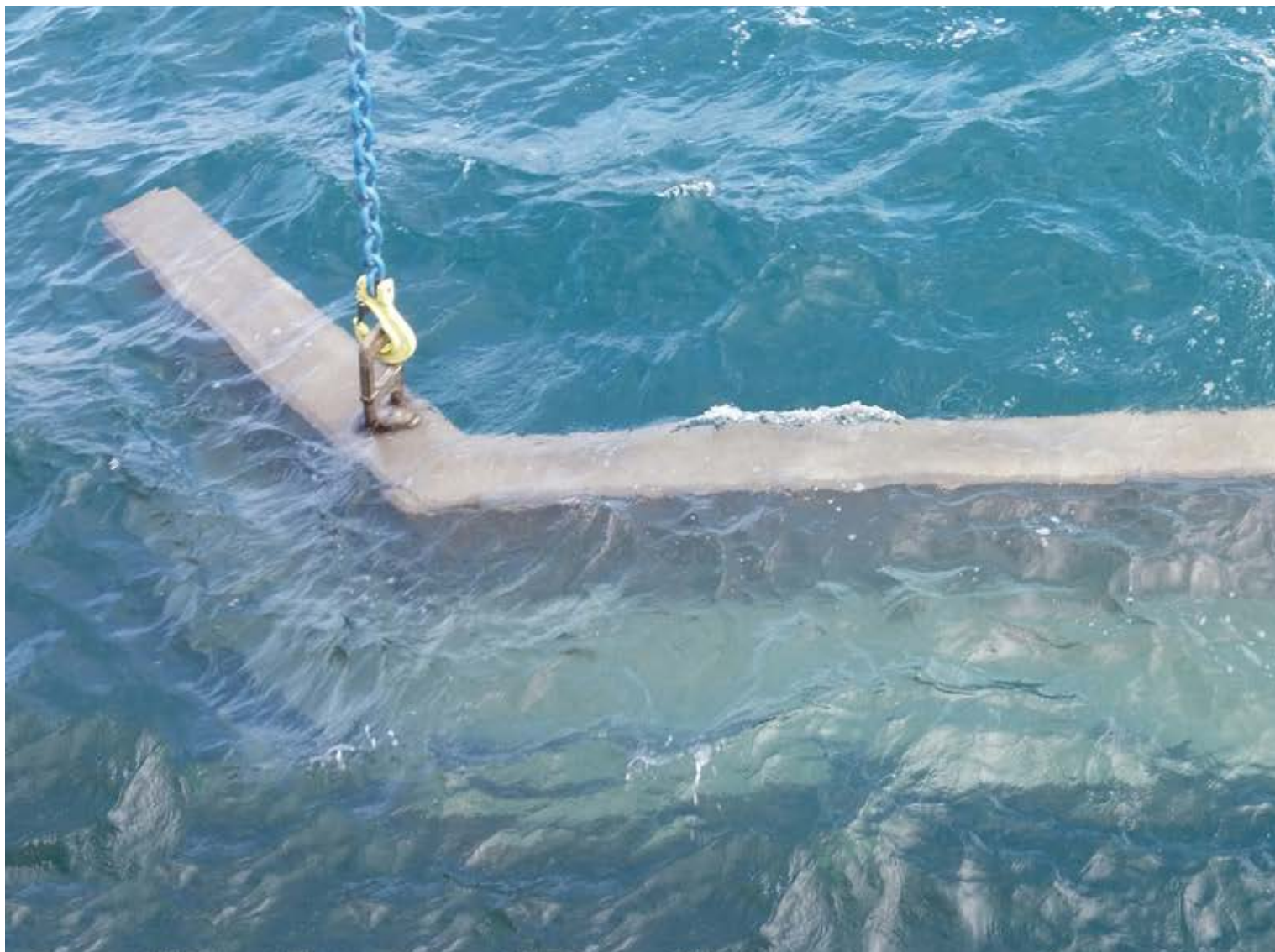
Divers precisely placed 17 precast pieces underwater to build the water crib.
