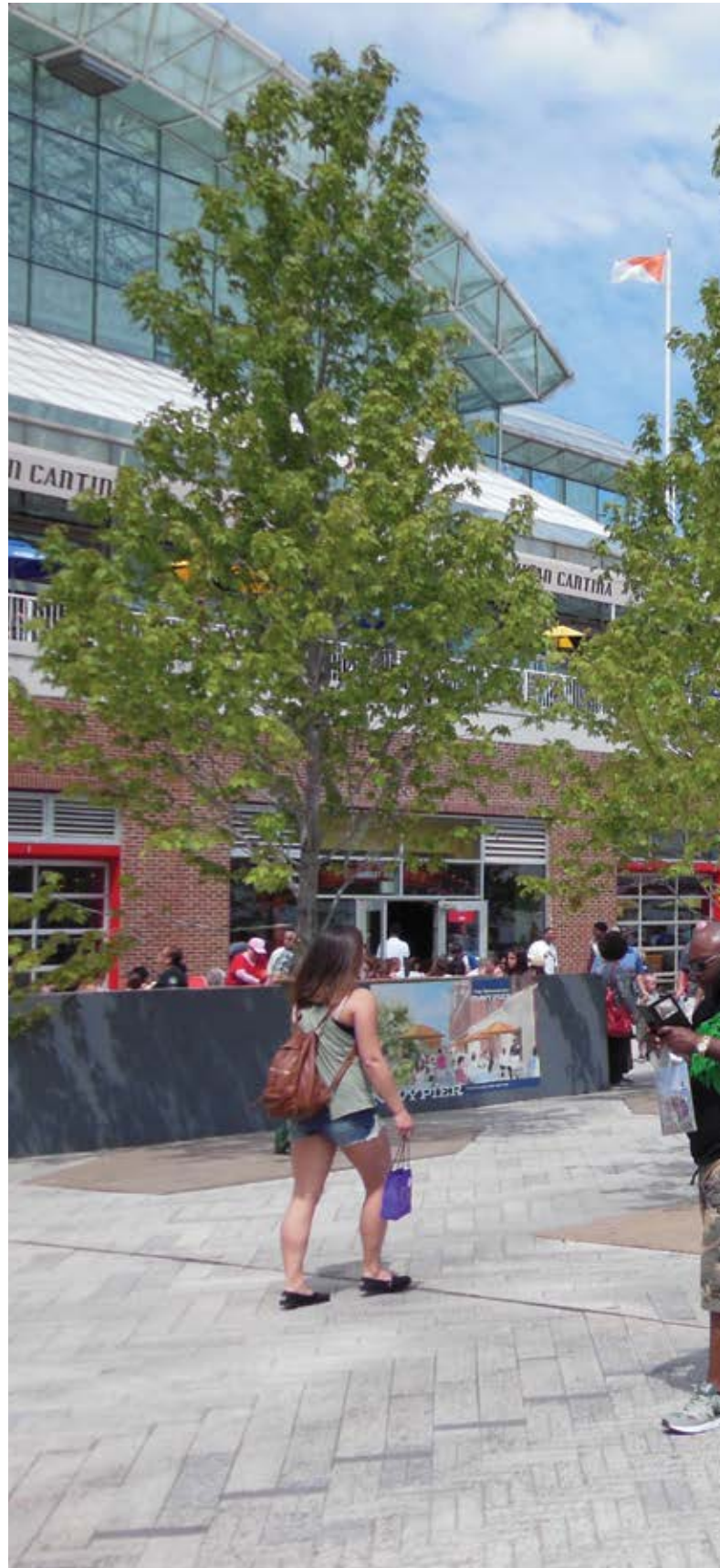
The installation of 59 massive precast concrete tree pits helps enhance the visitor experience at Chicago’s Navy Pier.
