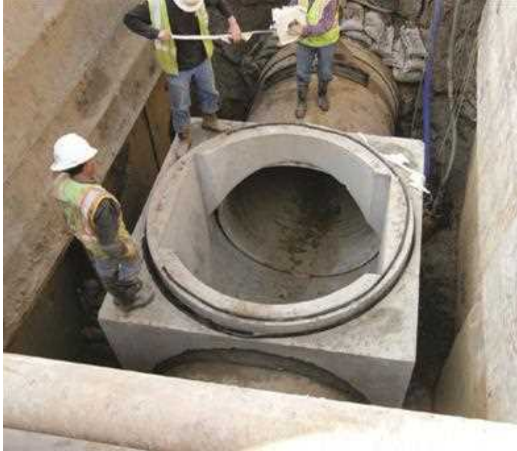
The Tindall T-Series Manholes address large diameter sewer installations.
