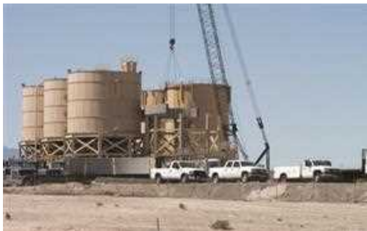
Olson Precast constructed and installed these precast silo supports in Las Vegas.
