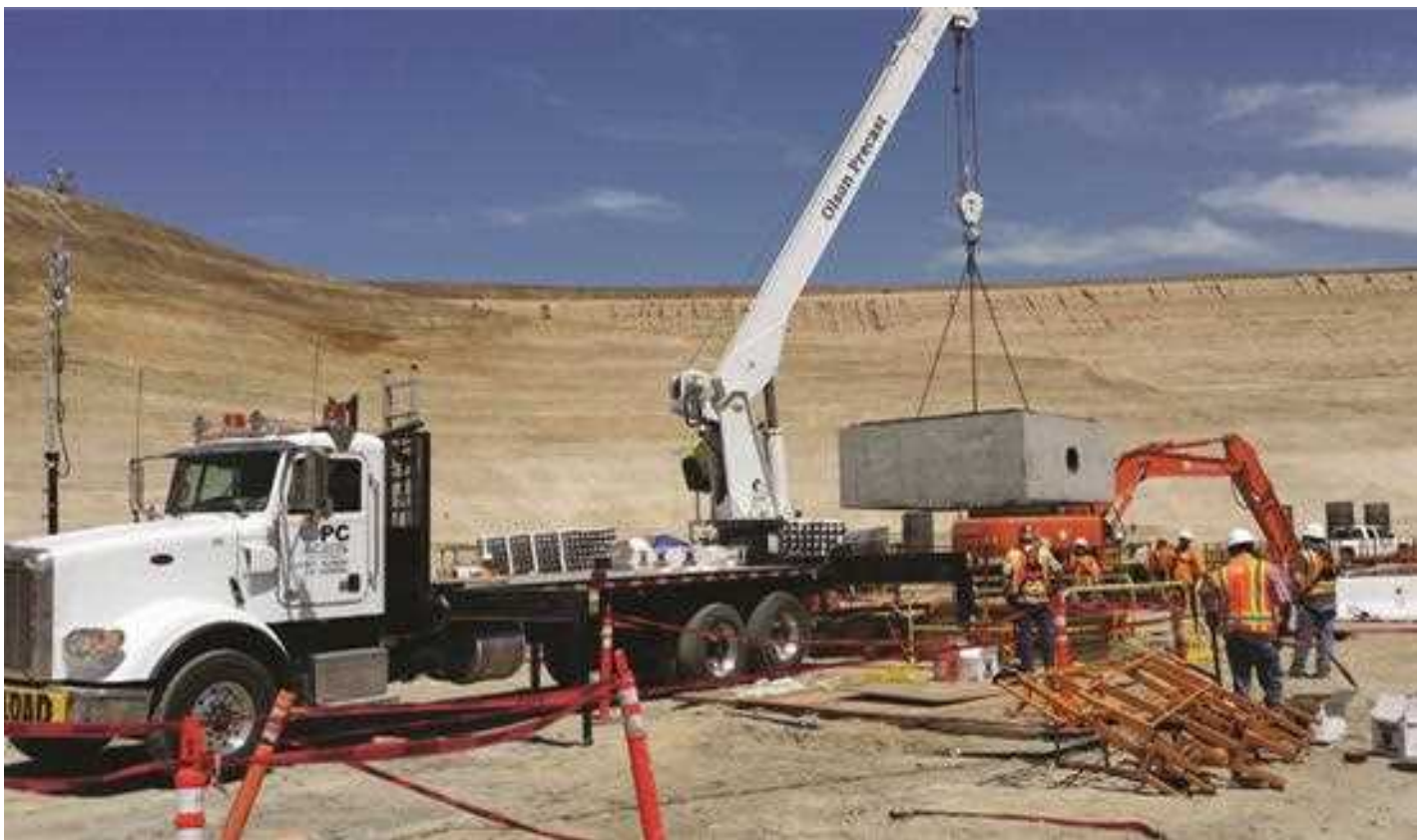
Olson Precast’s California facility constructed and installed sewage pumps and sewage ejector vaults for SoFi Stadium in Inglewood, Calif., home of the Los Angeles Rams, Los Angeles Chargers and Super Bowl LVI.
