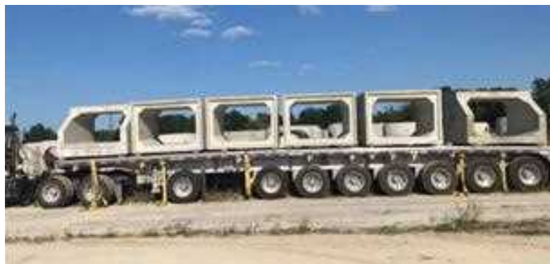
An entire box culvert run from Mack Industries is transported in one load.
