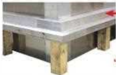
Pallet Forms placed on Riser Forms.
