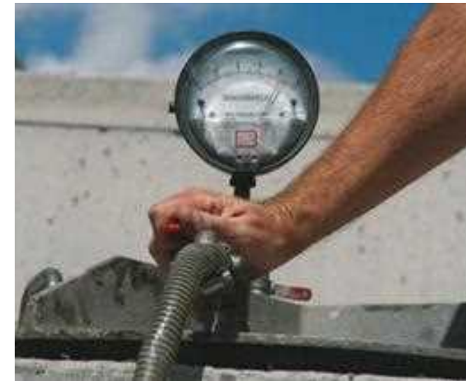
A tank is considered to have passed the vacuum test if the pressure is held at 4 inches Hg for a duration of 5 minutes.
