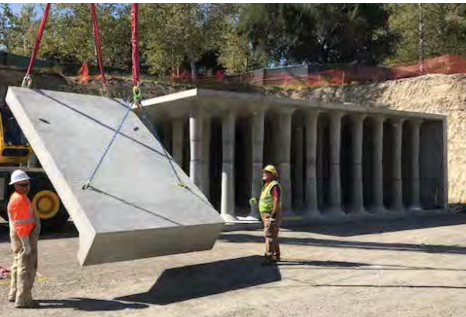
Workers install a massive precast concrete stormwater detention system in Gates Canyon Park, Calif. More than 270 precast pieces were used for the project.
